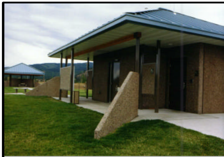
Non-Interstate Rest Area at Clearwater Junction - built in 1998
