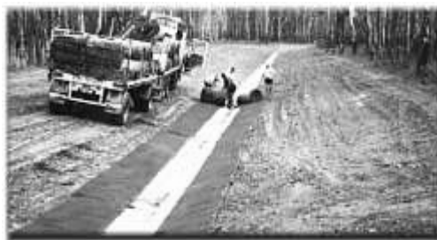
Figure 11. Sod placed in channel for erosion control in Australia (Jimboomba Turf Group)
