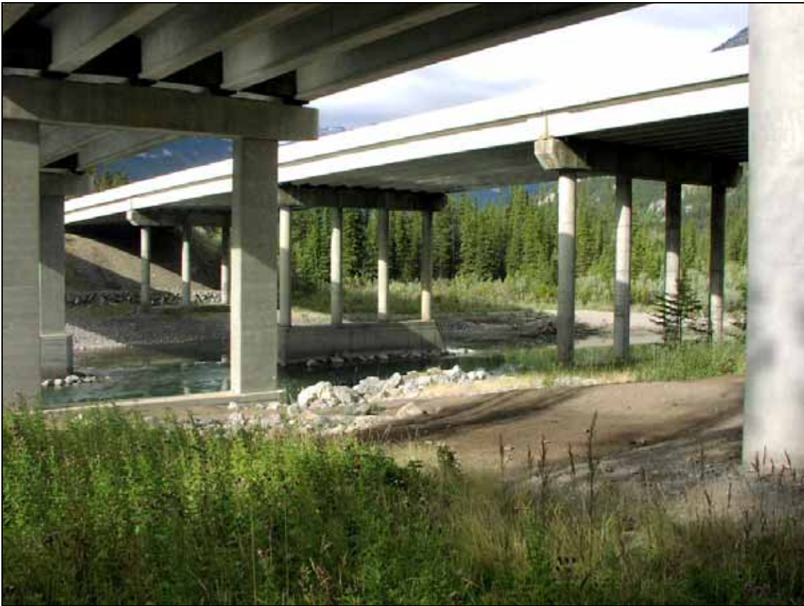
Figure 41. Photo. Viaduct with retention of riparian vegetation (Credit: Tony Clevenger).
