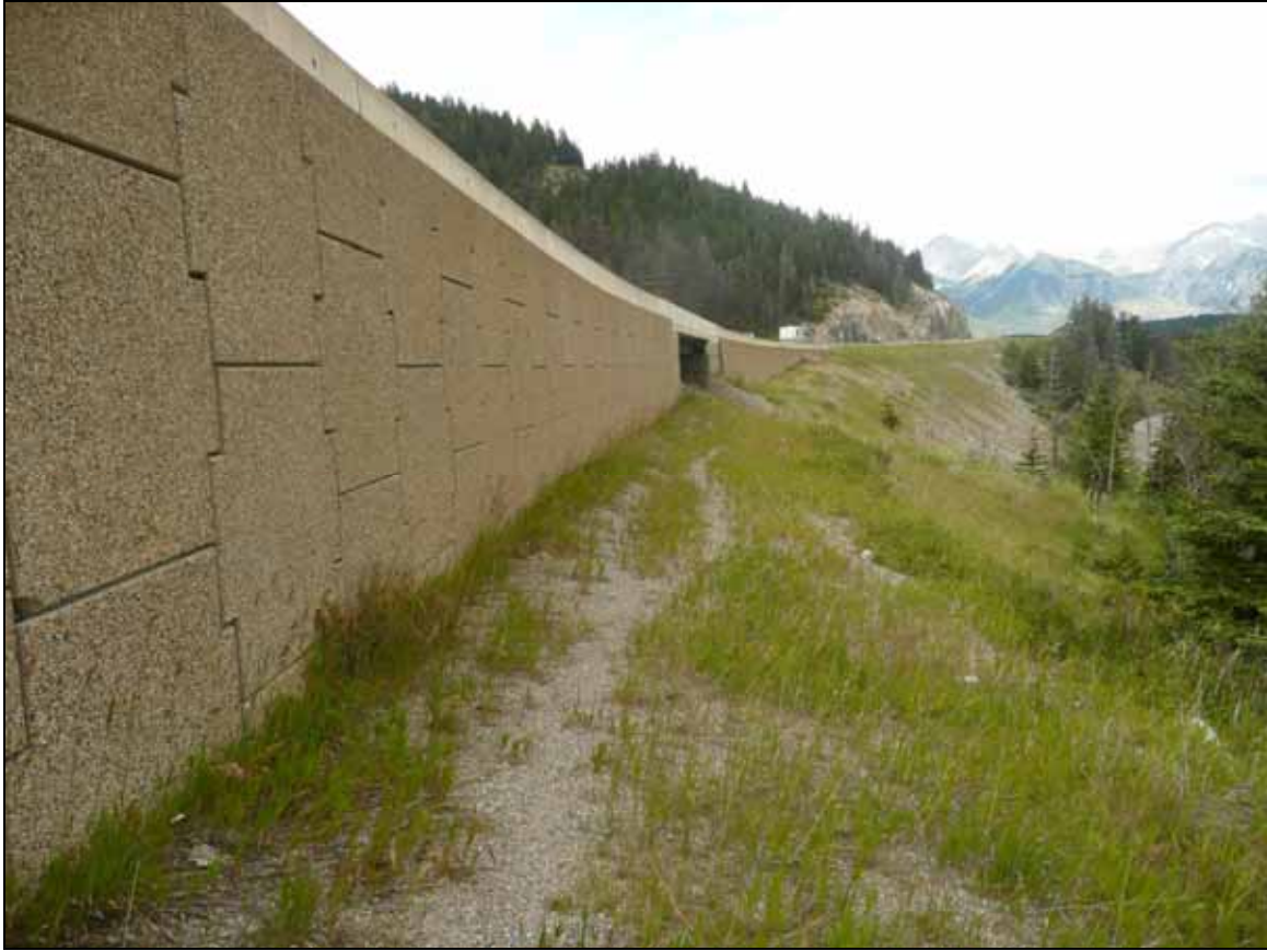
Figure 47. Photo. Mechanically stabilized earth (MSE) wall serving as wildlife exclusion “fence” (Credit: Tony Clevenger).
