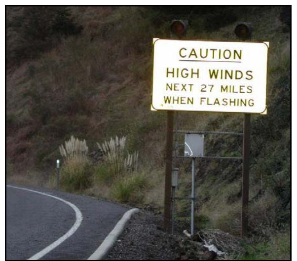
Figure 2-1: Static Sign with Flashing Beacon at Gold Beach
