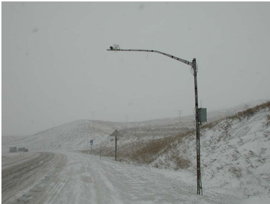
Figure 1-2: IceSight Installation on Roadway Shoulder
