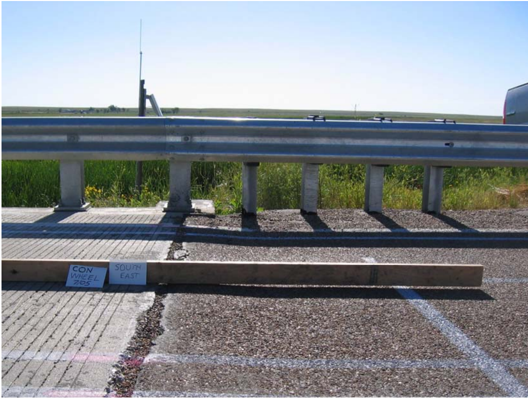
Figure H -9: Paved Approach – Southeast End of Conventional Deck
