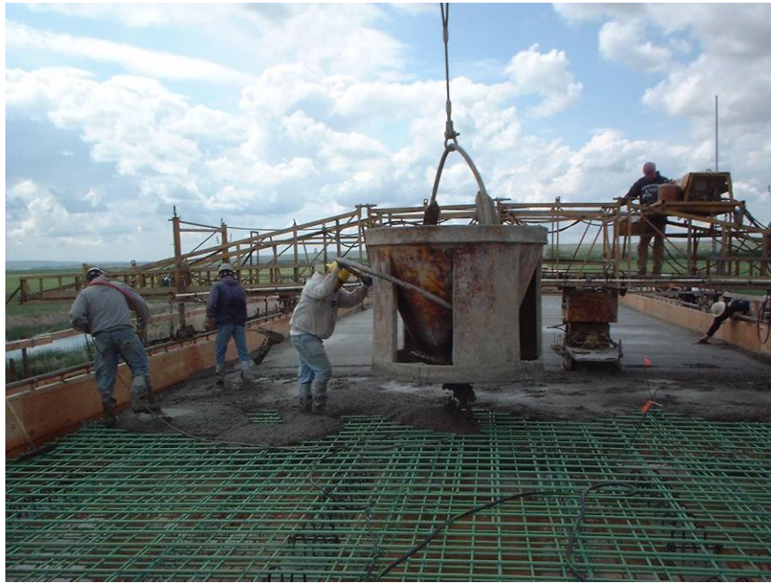
Figure 10: Placing the Deck Concrete
