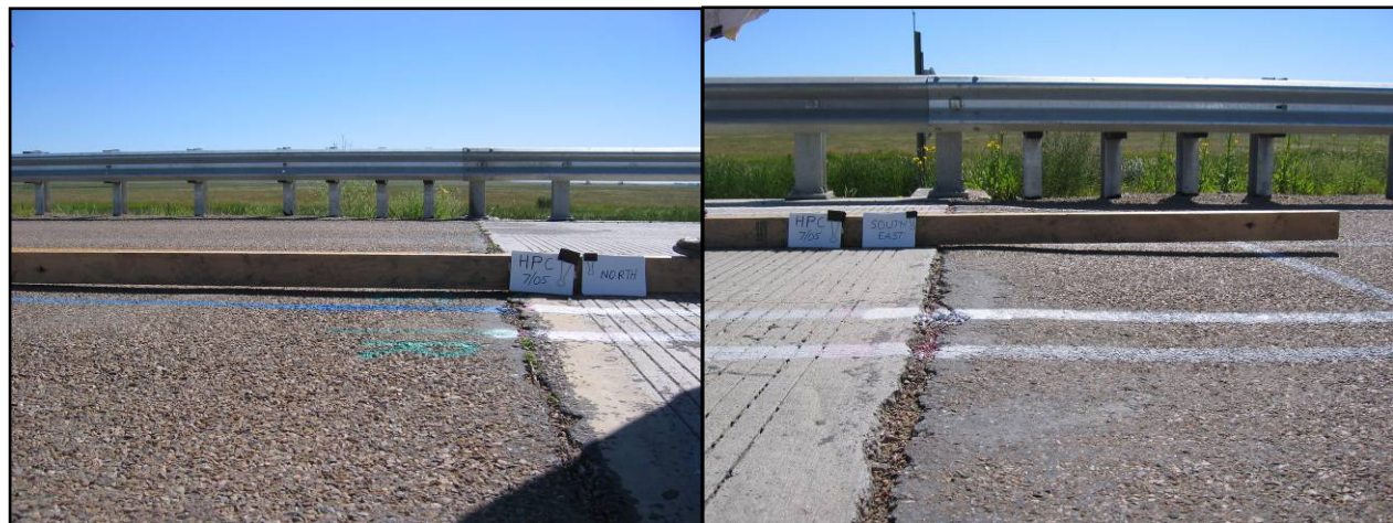
Figure 116: Paved Approaches of the HPC Deck (NW-left, SE-right)
