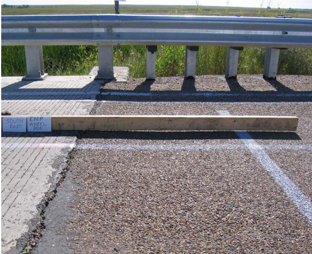
Figure H -22: Paved Approach – Southeast End of Empirical Deck
