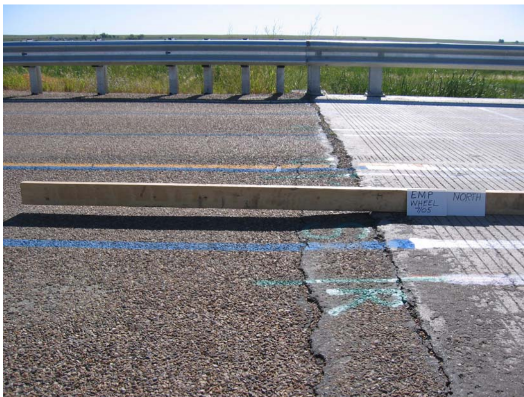
Figure H -21: Paved Approach – Northwest End of Empirical Deck
