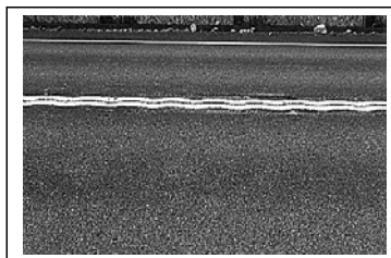
Figure 2 Centerline Rumble Strip
