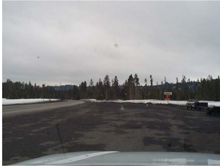
Figure 4: Example of Distance from Traveled Way
