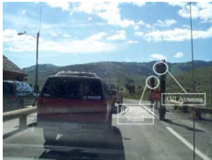
Figure 8: Antenna and Traffic Signal at North Entrance
