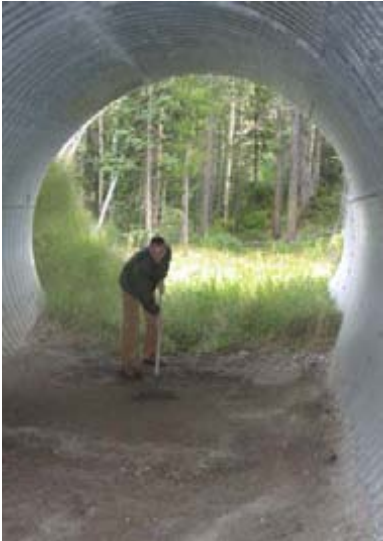
Exhibit 12-2: Raking of track bed in culvert, Banff National Park, Alberta (Source: T Clevenger/WTI).
