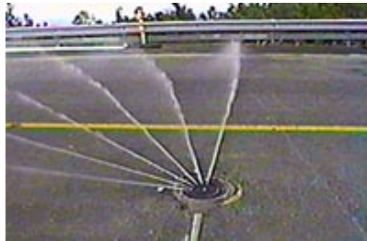
Figure 27: A FAST System in Action (Graphic Courtesy of the Ontario Ministry of Transportation).
