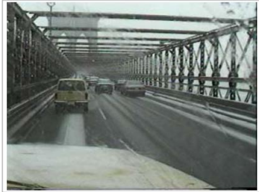
Photo Exhibit A: Pavement condition of roadway section sprayed with FAST system (3/14/99)
