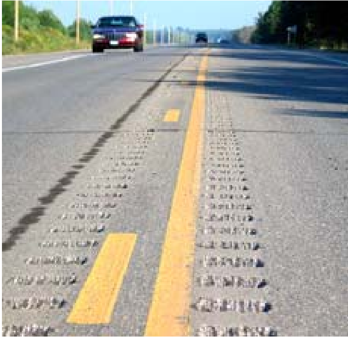
Figure 44: Centerline rumble strips. Photo by Minnesota Department of Transportation.
