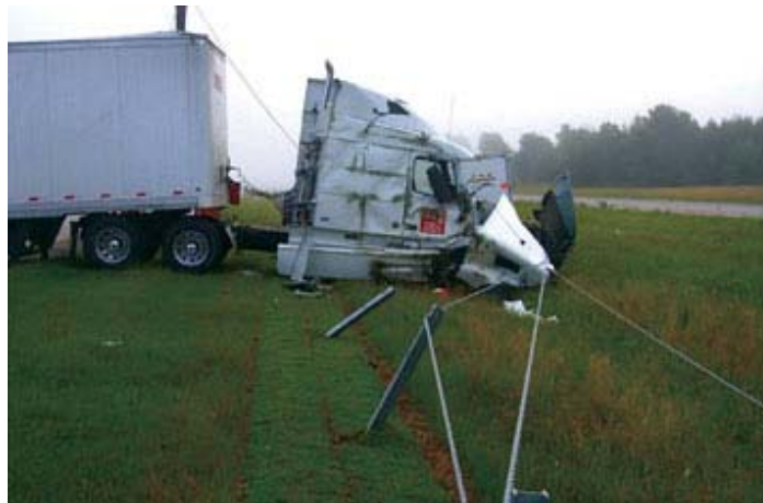
Figure 43: Cable median barrier. Photo courtesy of NCDOT.
