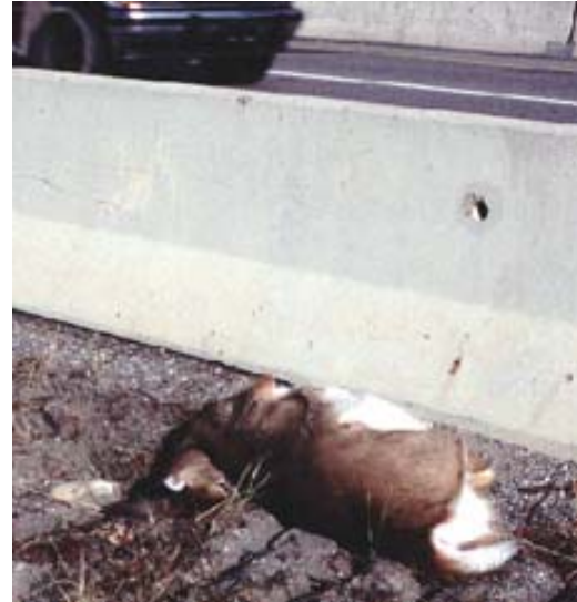
Figure 39: Solid concrete barrier with white-tailed deer carcass. Photo by A. P. Clevenger.
