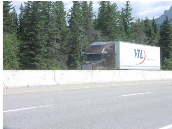
Figure 37: Solid continuous concrete barrier. Photo by A. P. Clevenger.
