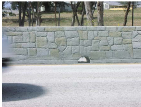
Figure 1: Caltrans included basal openings in the Highway 1 concrete barrier for small animal passage. Photo by A.P. Clevenger
