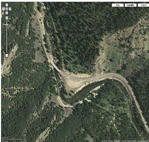
Figure 2: A 35 MPH Bridge over Gallatin River (courtesy Google Imagery).
