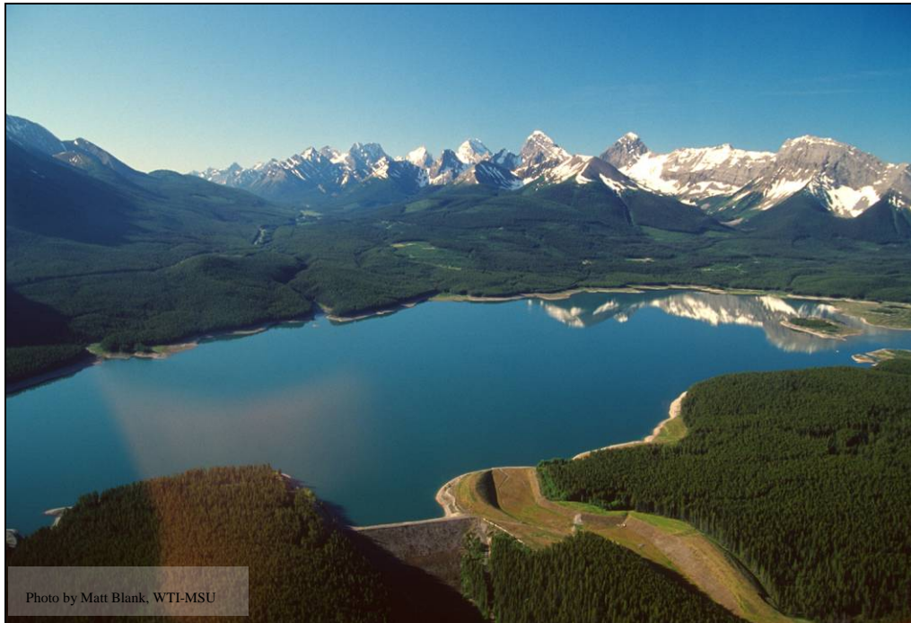
Figure 9: Canyon Dam located on the Spray River System, a major tributary watershed to the Bow River in Reach 3. Prior to construction, the Spray River flowed through the channel outlined in the foreground. Currently, 75% of the water is directed toward Canmore.
