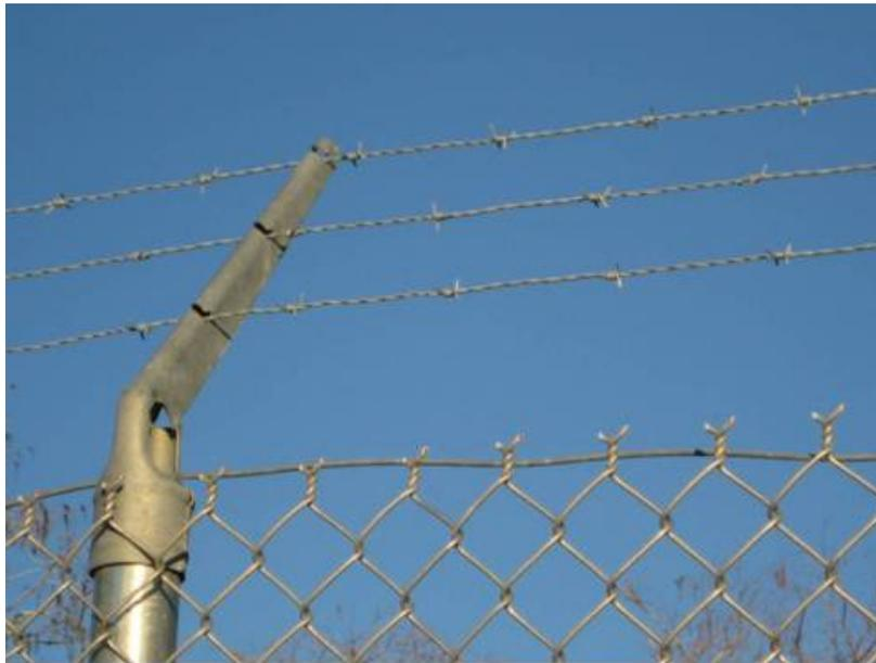
**Figure 17. A 3.4-m-high (11-ft-high) chain-link fence along SR 29 in southern Florida equipped with three strands of outrigged barbed wire to prevent Florida panthers from climbing the fence (copyright: Marcel Huijser).**
