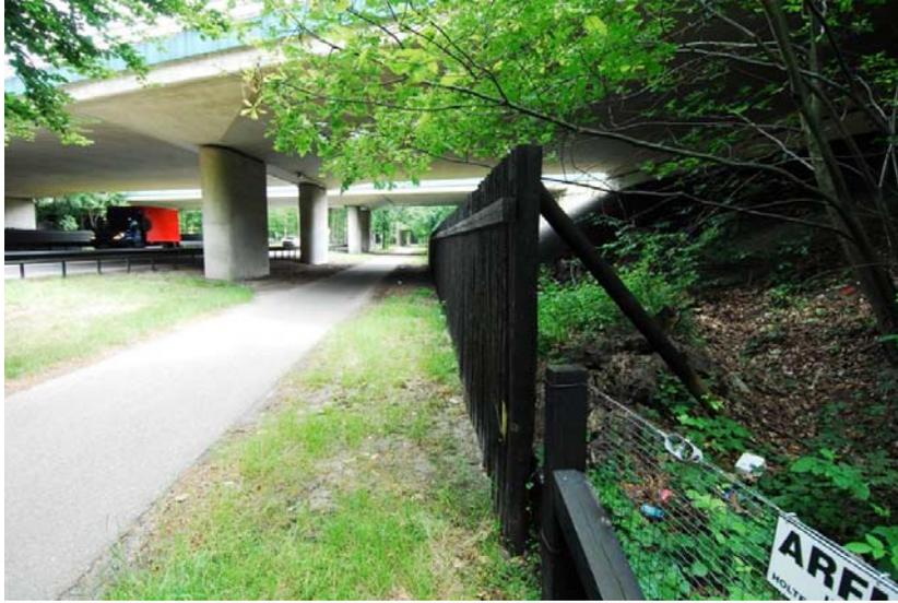
**4** Figure 83. An underpass for a road (Hilversumsestraatweg) under the motorway A27 near the town "Hilversum", The Netherlands, that was modified with soil and tree stumps to encourage co-use by wildlife to the right of the fence. The purpose of the fence, which is painted black, is to reduce light and noise disturbance from traffic (copyright: Marcel Huijser).
