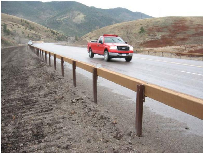
**Figure 7. Example of box beam guardrail (copyright: Marcel Huijser).**
