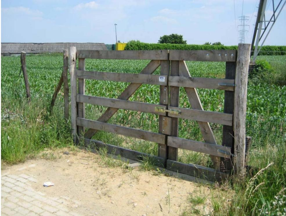
**Figure 127.** A gate that allows for access to a field with crops through an amphibian barrier, and a medium- and large-mammal fence, near wildlife overpass "Schinheugel," near the town Roermond, The Netherlands. Note that the gate connects closely to a hard surface to prevent amphibians and other small species from entering the road corridor. (copyright: Marcel Huijser).
