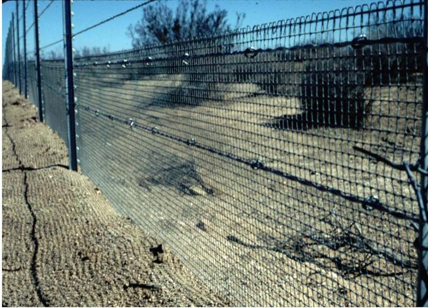
**Figure 107. Tortoise barrier fence erected along State Highway 58 near Kramer Junction, San Bernardino County, CA (copyright: William I. Boarman, U. S. Geological Survey).**
