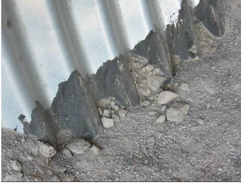
**Figure 55. Soil in corrugated metal culvert makes it more suitable for use by wildlife (copyright: Marcel Huijser).**
