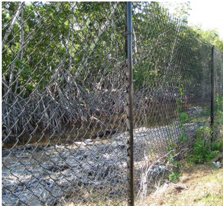
Figure 31: A 1.83 m (6 ft) high chain link fence along U.S. Hwy 1 between Florida City and Key Largo, Florida, has been coated with plastic to make the fence blend in with its surroundings (© Marcel Huijser).
