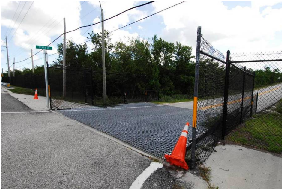
Figure 45: Wildlife guard along U.S. Highway 1 for Key deer on Big Pine Key, Florida (© Marcel Huijser).
