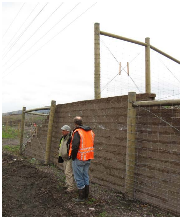
Figure 38: A jump-out along a 2.4 m (8 ft) high fence along U.S. Highway 93 in Montana (© Marcel Huijser).
