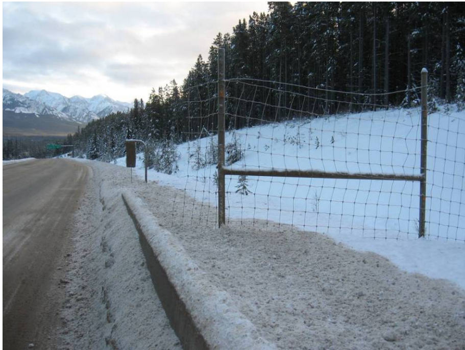
Figure 37. Fence end brought close to the road with a concrete barrier for safety along Hwy 93S in Banff National Park, just west of Castle Jct (© Marcel Huijser, WTI-MSU).
