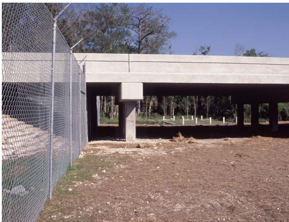
Figure 51: Underpass in southern Florida that allows for ecosystem processes (hydrology) as well as wildlife use, including the Florida Panther (© Marcel Huijser).
