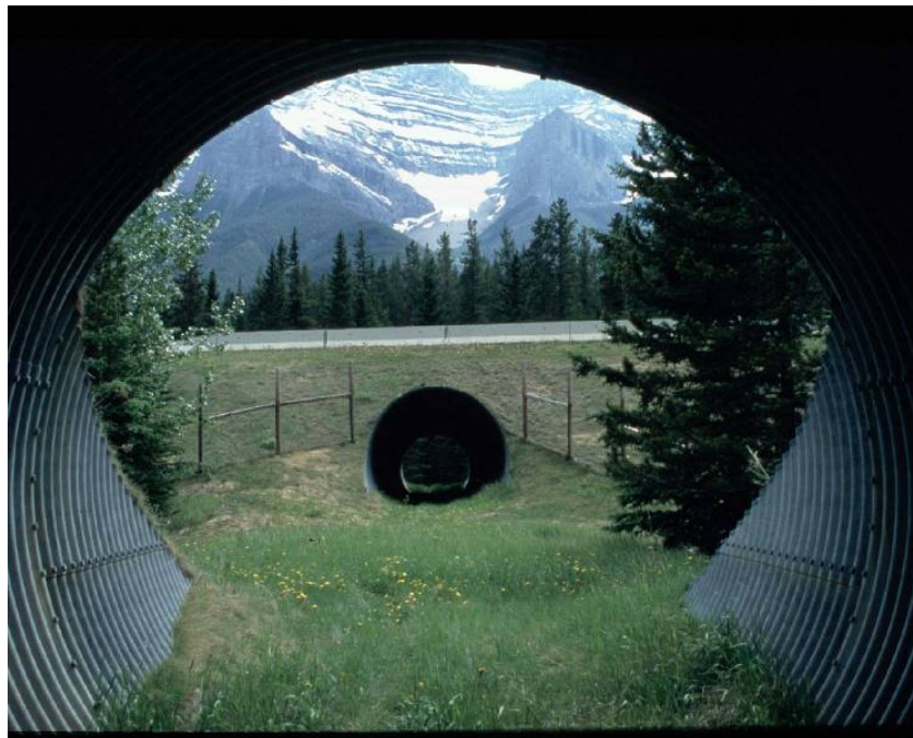
Figure 48: A large wildlife crossing culvert along the Trans-Canada Highway in Banff National Park, Alberta (© Tony Clevenger).
