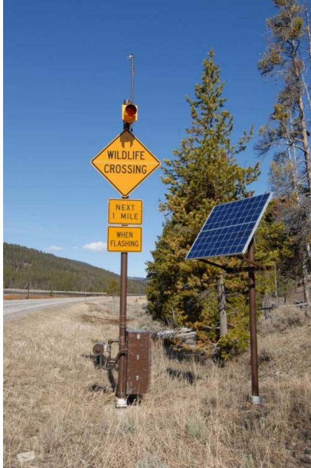
Figure 4: An animal detection system on U.S. Highway 191 in Yellowstone National Park (© Marcel Huijser).
