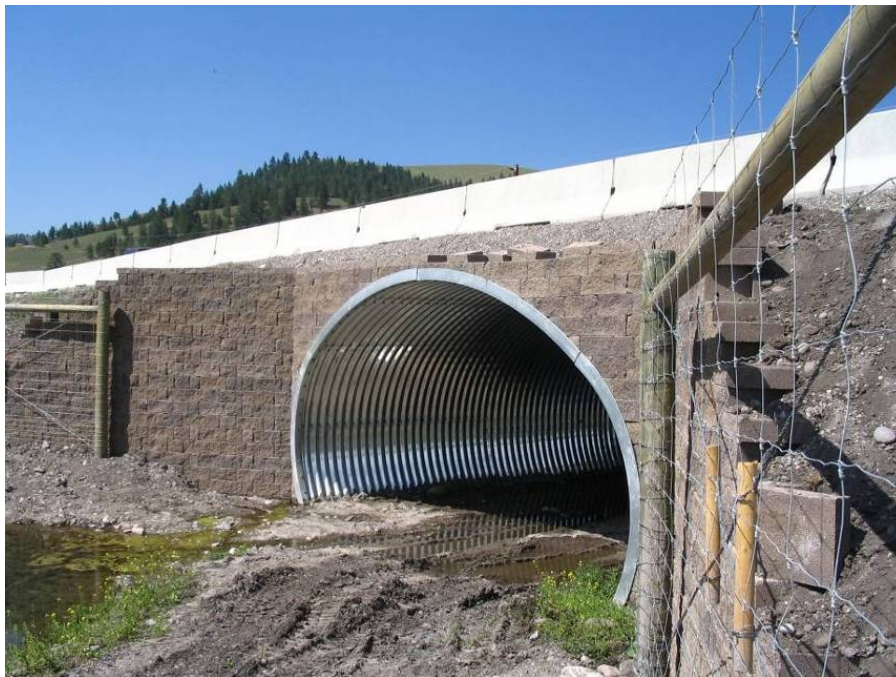
Figure 50: Wildlife underpass along U.S. Highway 93 on the Flathead Indian Reservation, Montana (© Marcel Huijser).
