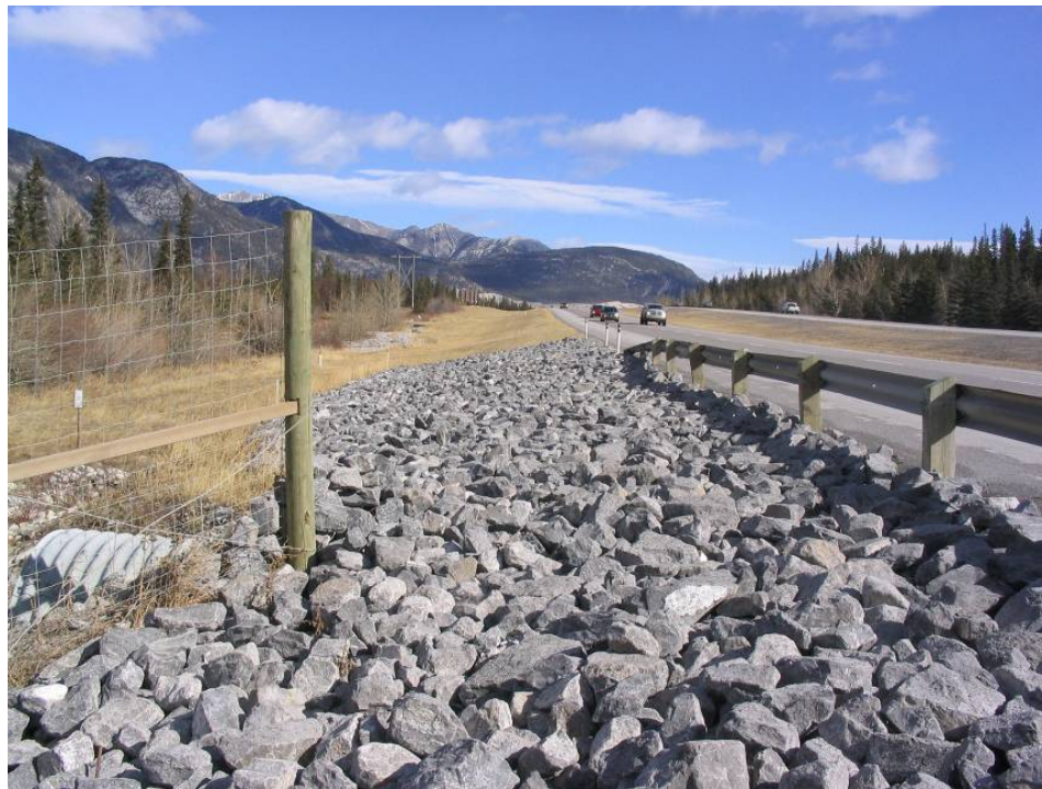
Figure 36: The boulder field at the fence end at Dead Man's Flats along the Trans-Canada Highway east of Canmore, Alberta (© Bruce Leeson).
