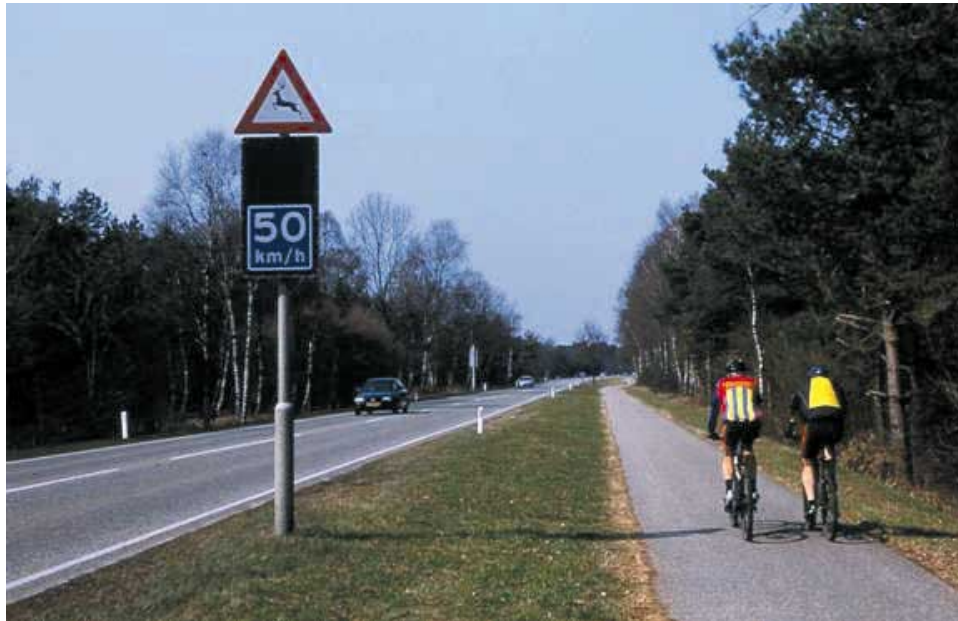
Figure 9: Advisory speed limits accompany a deer warning sign near ‘t Harde, The Netherlands (© Marcel Huijser). Note: The LED part of the warning sign is linked to an animal detection system, but the advisory speed limit reduction sign is always visible in daylight, regardless of the presence and detection of large animals.
