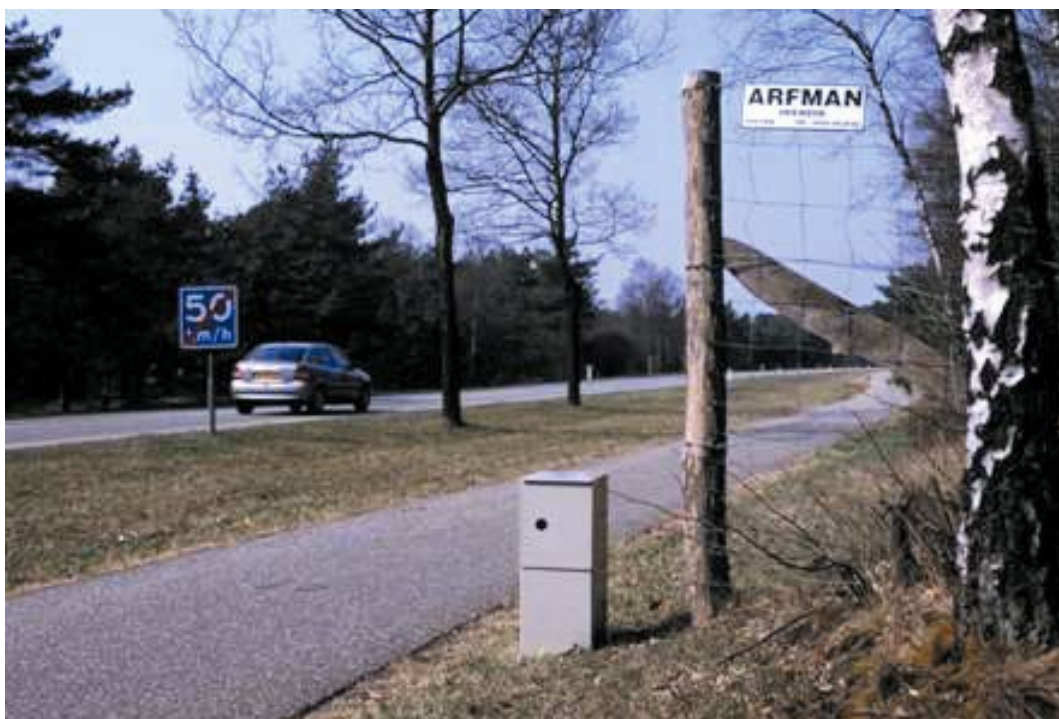
Figure 35: Gap in a wildlife fence combined with an animal detection system, wildlife warning signs and advisory speed limit reduction, the Netherlands (© Marcel Huijser).
