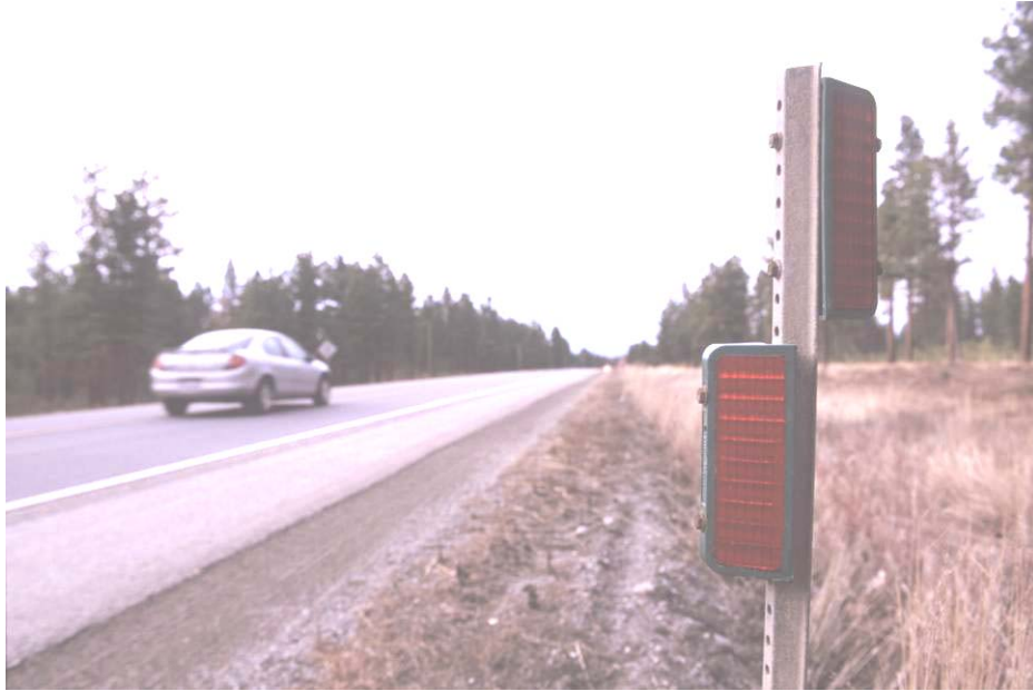
Figure 25: Deer reflector along Hwy 93 in British Columbia (© Marcel Huijser).
