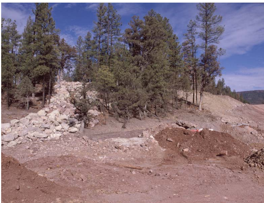
Figure 33: Large boulders placed in the right-of-way as a barrier to elk and deer with a view of State Route 260 (under construction) in Arizona (© Marcel Huijser).
