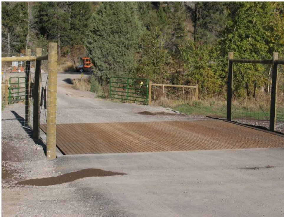
Figure 44: Wildlife guard along U.S. Highway 93 on the Flathead Indian Reservation, Montana (© Marcel Huijser).
