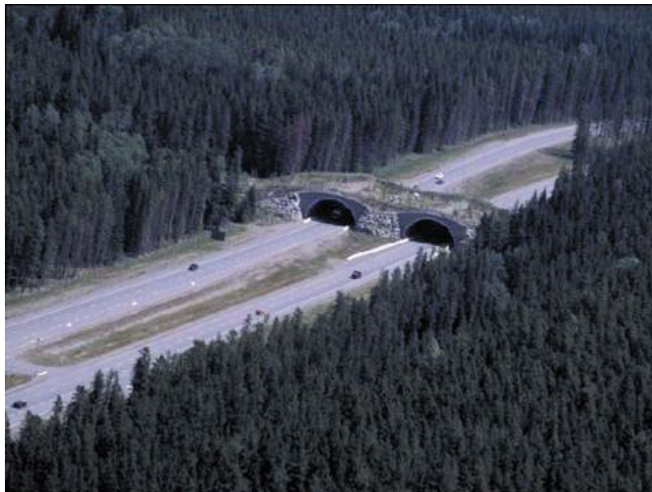
Figure 47: Red Earth Overpass on the Trans-Canada Highway (© Tony Clevenger).
