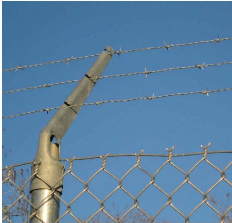
Figure 29: A 3.4 m high chain link fence along SR 29 in southern Florida was equipped with three strands of outriggered barbed wire to prevent Florida panthers from climbing the fence (© Marcel Huijser).
