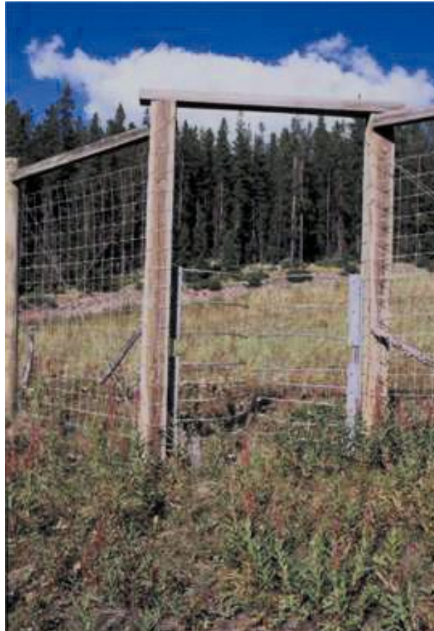
Figure 41: One-way elk gate in British Columbia, (© Marcel Huijser).
