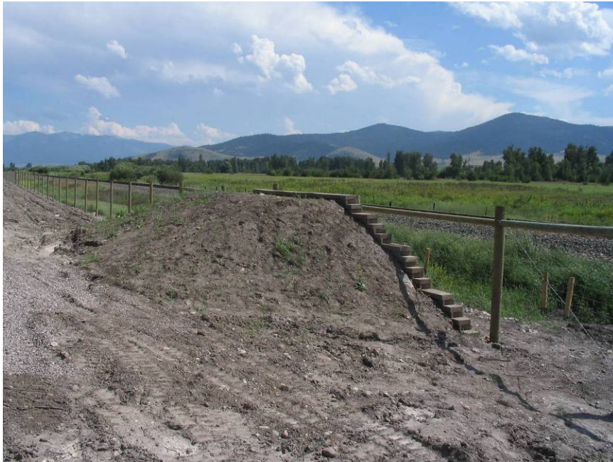
Figure 38: A jump-out along a 2.4 m (8 ft) high fence along U.S. Highway 93 in Montana (© Marcel Huijser).
