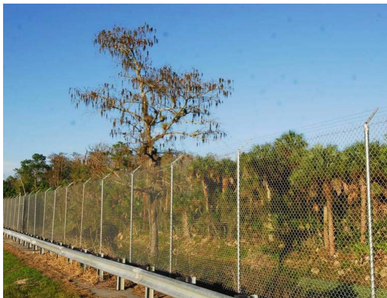
Figure 28: A 3.4 m high chain link fence along SR 29 in southern Florida designed to prevent Florida panthers from entering the roadway and to guide them toward underpasses (© Marcel Huijser).
