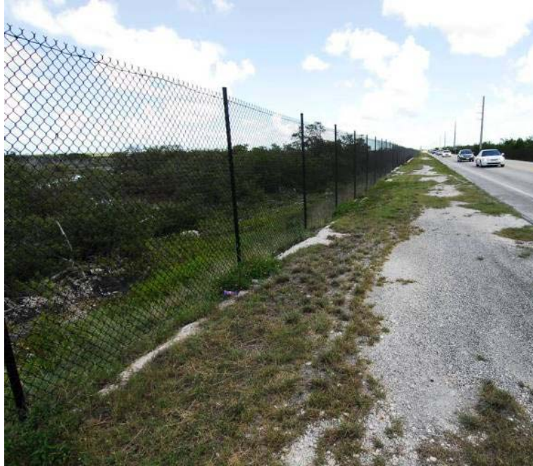
Figure 30: A 2.44 m (8 ft) high chain link fence along U.S. Hwy 1 on Big Pine Key, Florida, has been coated with plastic to make the fence blend in with its surroundings (© Marcel Huijser).
