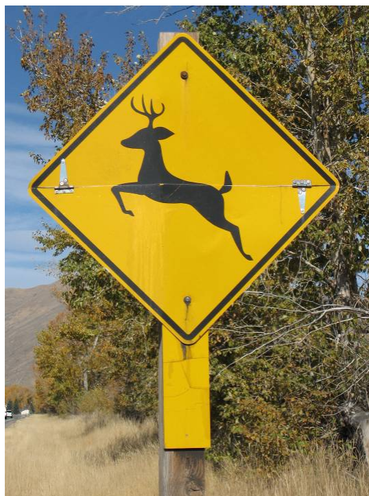
Figure 21: A permanent deer warning sign in Idaho has hinges, allowing for its seasonal use (© Marcel Huijser).
