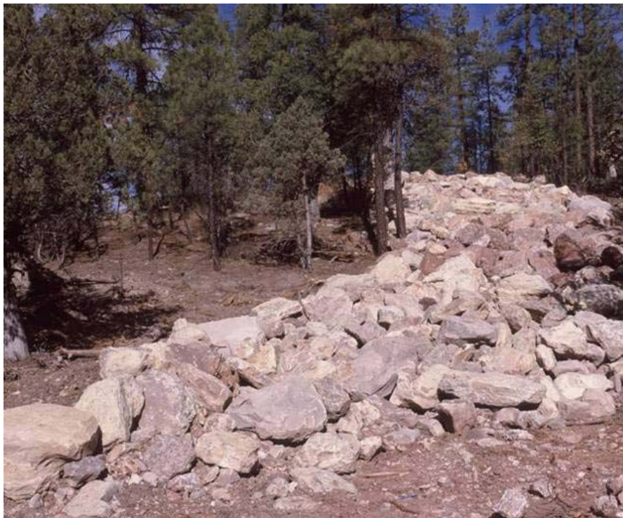
Figure 32: Large boulders placed in the right-of-way as a barrier to elk and deer along State Route 260 in Arizona (© Marcel Huijser).
