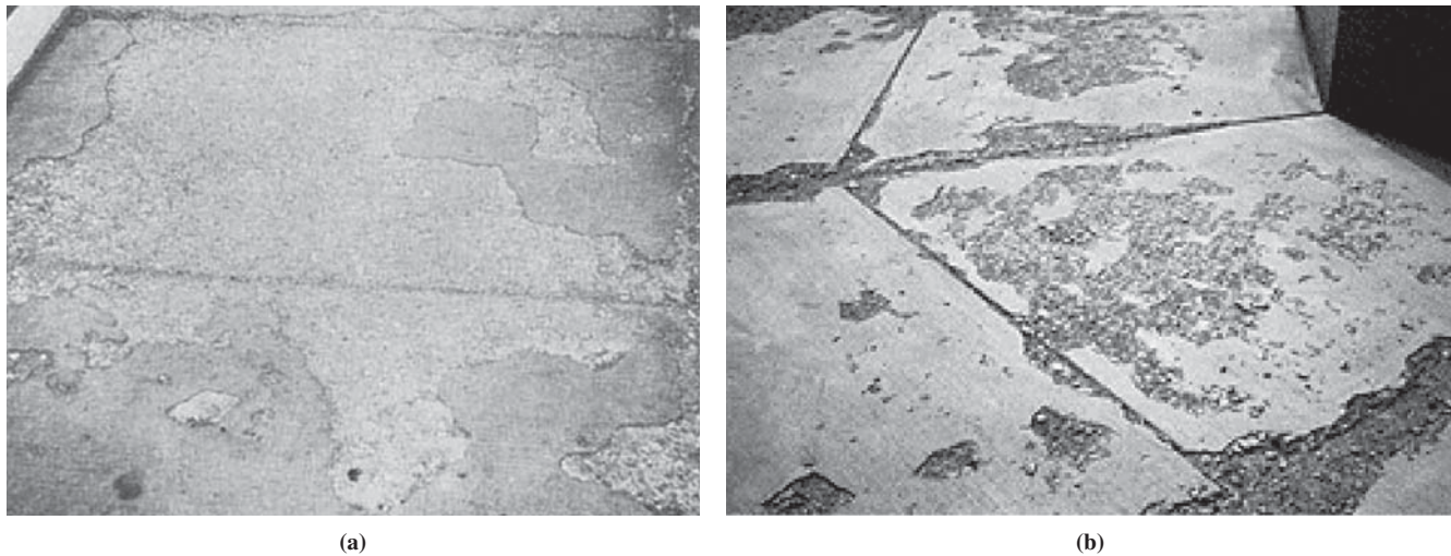
FIGURE 14 Concrete scaling (a) and spalling (b) [adapted from Potomac Construction Industries (2007) and Cryotech Deicing Technology (2007), respectively].
