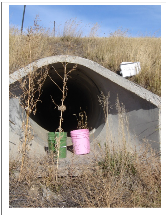
Figure 13. View of R351.2 entrance (152 cm [60 in] in diameter (left) and adjacent landscape (right).
