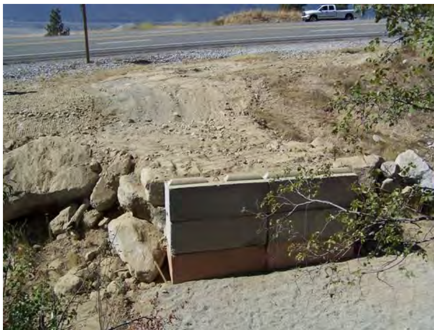
Exhibit 8. Escape ramps on US 95 near Bonners Ferry, Idaho. (a) Lateral view of escape ramp fitted into boulder wall on downhill side of highway; (b) elevated view of escape ramp under construction with landing pad in place. (copyright: Tony Clevenger [a] and Wayne Wakkinen [b])
