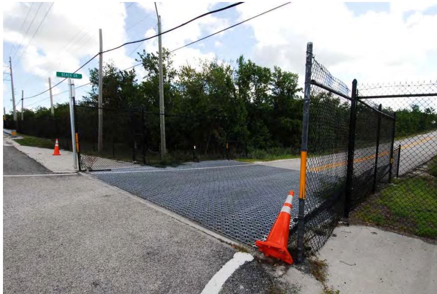
Figure 49: Wildlife guard along U.S. Highway 1 for Key deer on Big Pine Key, Florida (© Marcel Huijser).
