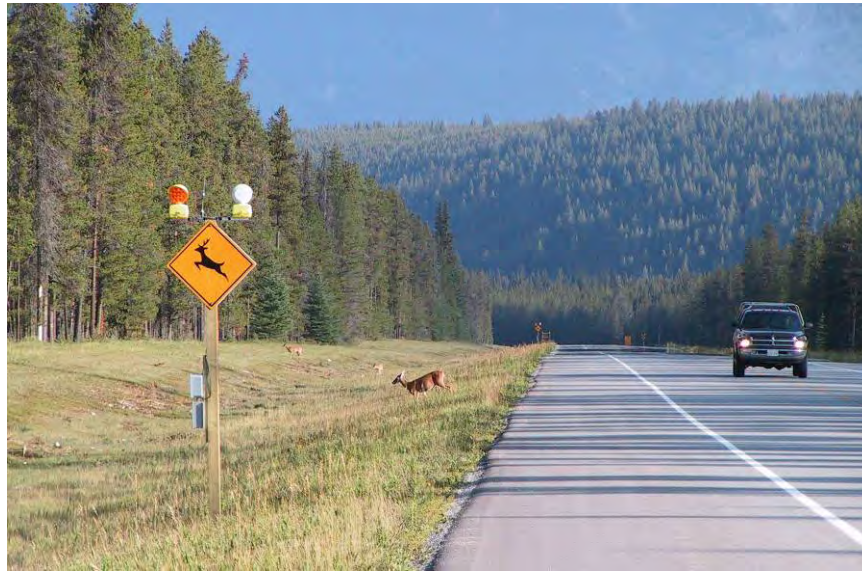
Figure 20: An animal detection system in action in Kootenay National Park, British Columbia (© Alan Dibb).
