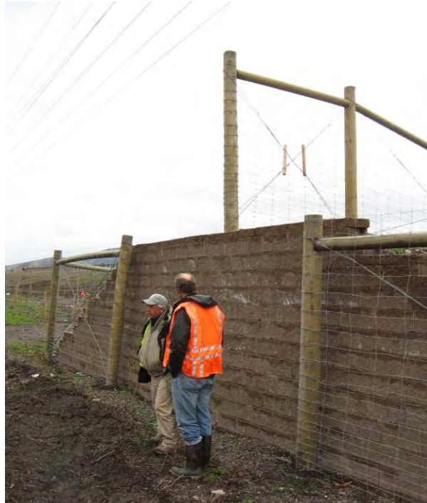
Figure 43: A jump-out along a 2.4 m (8 ft) high fence along U.S. Highway 93 in Montana (© Marcel Huijser).
