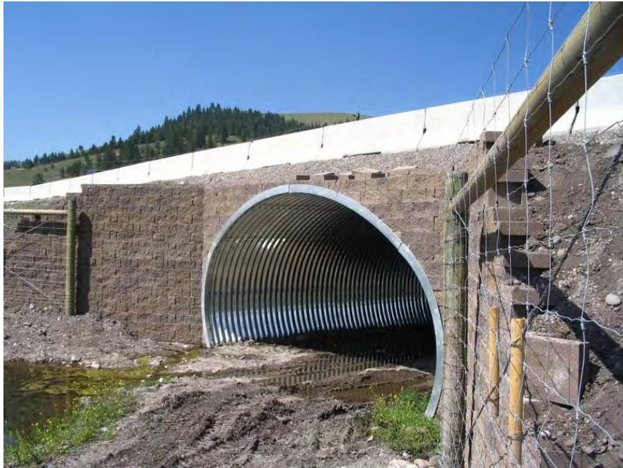
Figure 54: Wildlife underpass along U.S. Highway 93 on the Flathead Indian Reservation, Montana (© Marcel Huijser).
