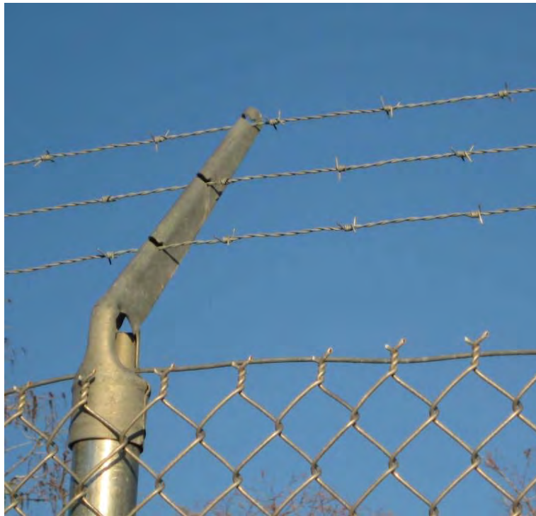
Figure 34: A 3.4 m high chain link fence along SR 29 in southern Florida was equipped with three strands of outriggered barbed wire to prevent Florida panthers from climbing the fence (© Marcel Huijser).
