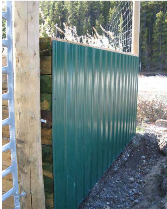
Figure 44: A jump-out along a 2.4 m (8 ft) high fence with smooth metal to prevent bears from climbing into the right-of-way along the Trans-Canada Highway, Lake Louise area, Banff National Park, Canada (© Marcel Huijser).
