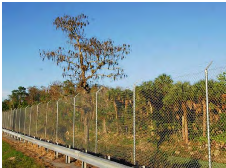
Figure 33: A 3.4 m high chain link fence along SR 29 in southern Florida designed to prevent Florida panthers from entering the roadway and to guide them toward underpasses (© Marcel Huijser).
