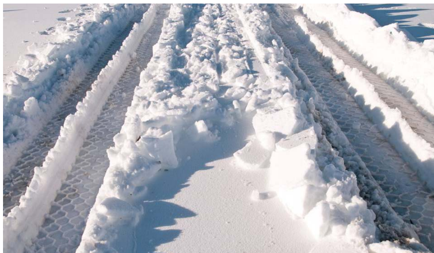
Figure 47: Deep snow compacted using the plow truck.
