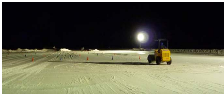
Figure 40: Compacting test sections with a smooth-drum compactor.
