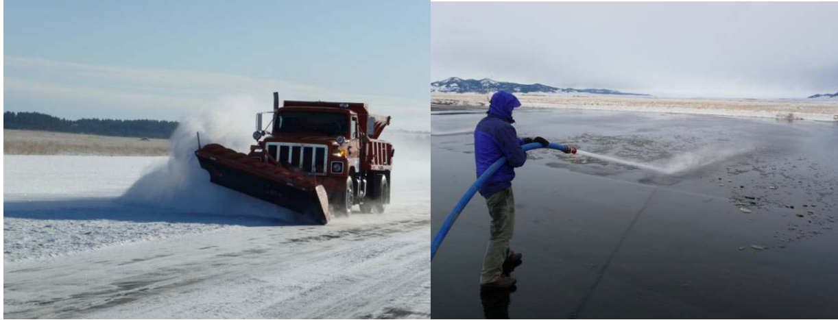
Figure 11 Clearing and washing test sections on the driving surface area using a plow truck and high pressure hose.
