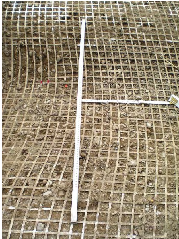
Figure 43. Example of horizontal distortion of a geosynthetic due to trafficking.
