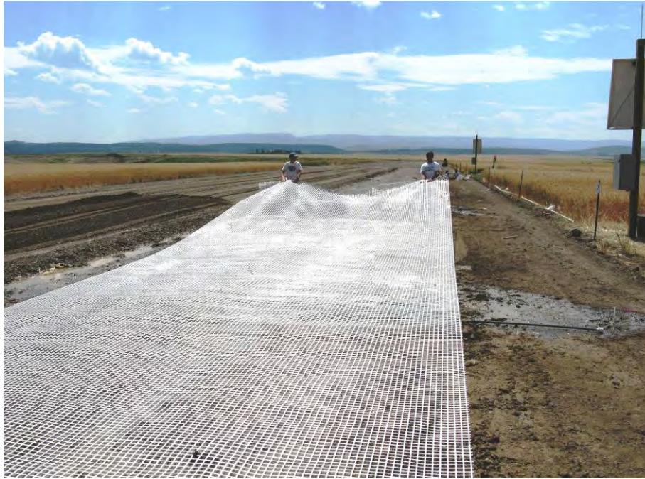
Figure 26. Installation of geosynthetics.
