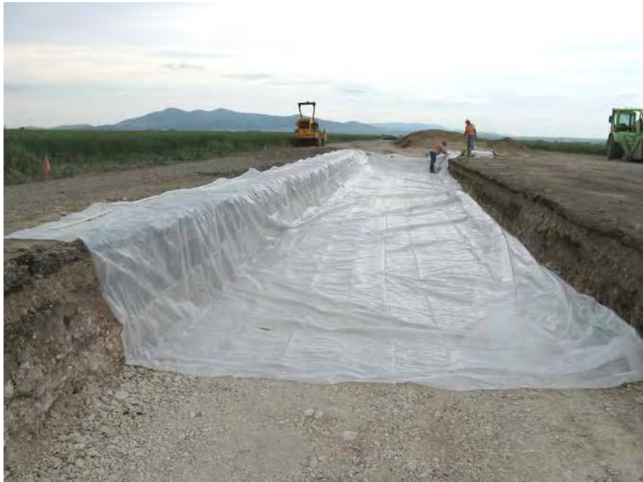
Figure 14. Installation of plastic liner in test pit.
