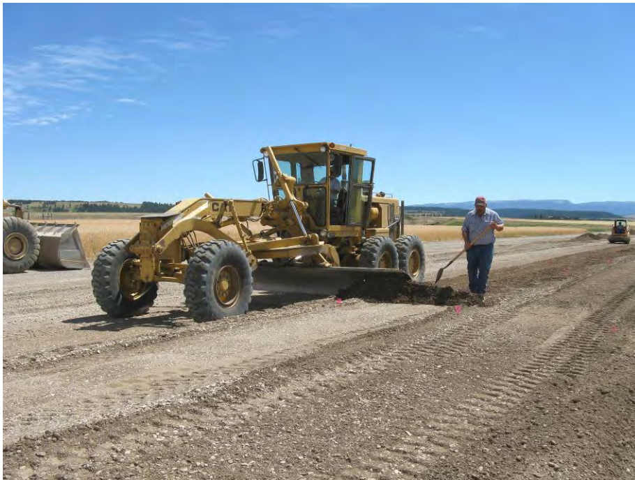
Figure 28. Final grading of the base course surface.
