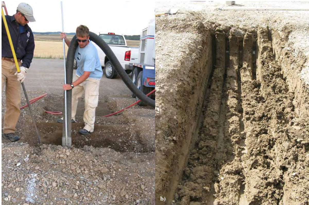
Figure 34. Forensic investigations: a) air and vacuum removal of base course, b) excavation of subgrade.
