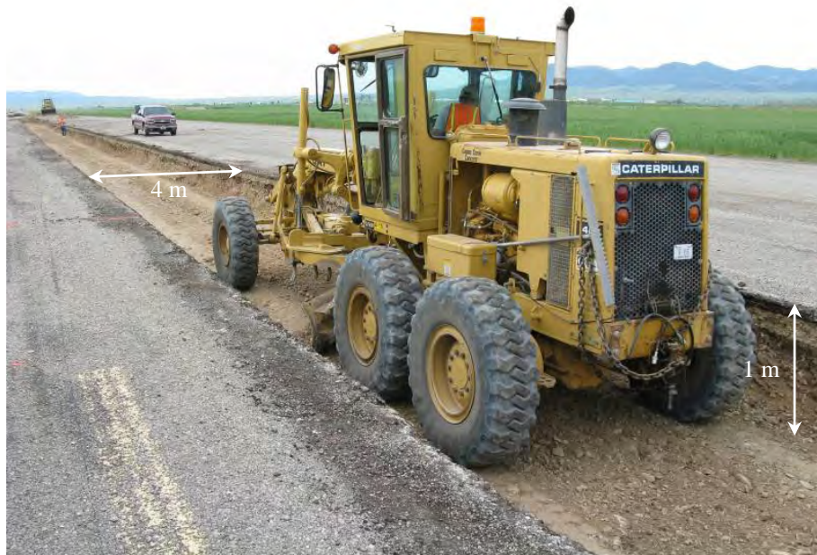
Figure 13. Final grading of the test pit.
