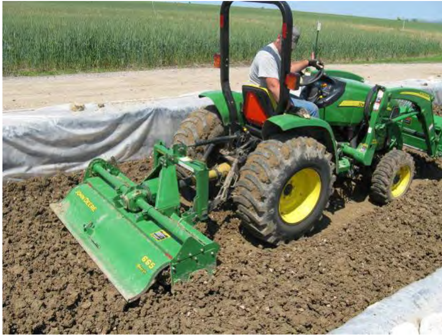
Figure 16. Mixing the subgrade layer with large roto-tiller.
