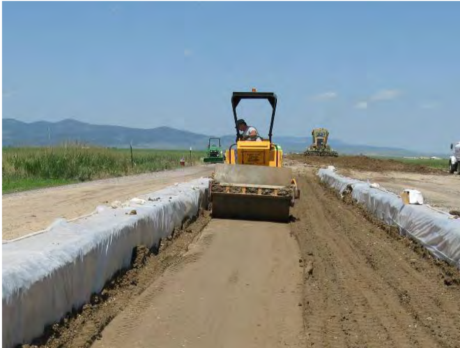
Figure 17. Compacting subgrade with smooth drum, vibratory roller.
