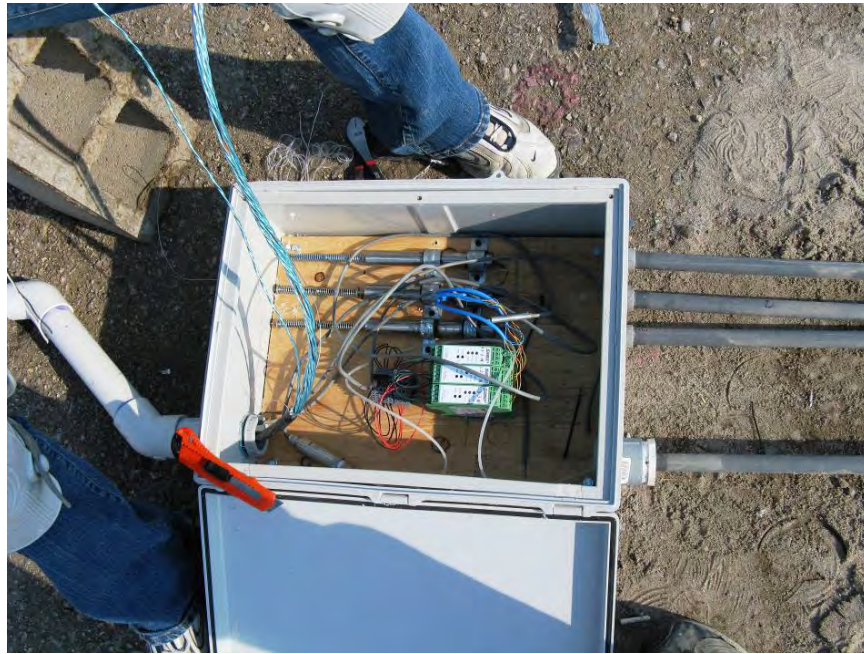
Figure 8. Installation of sensor box.
