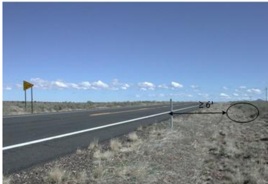
HAR Static Sign Placement on SR 64
