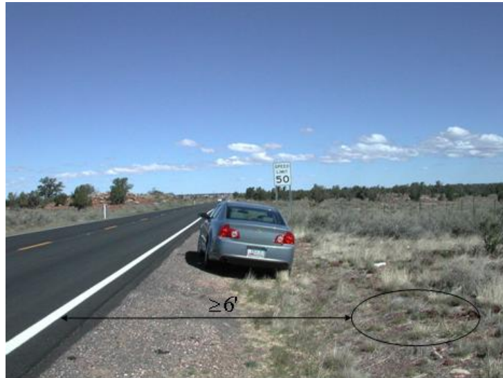
Figure 11: HAR Static Sign Location on US 180
