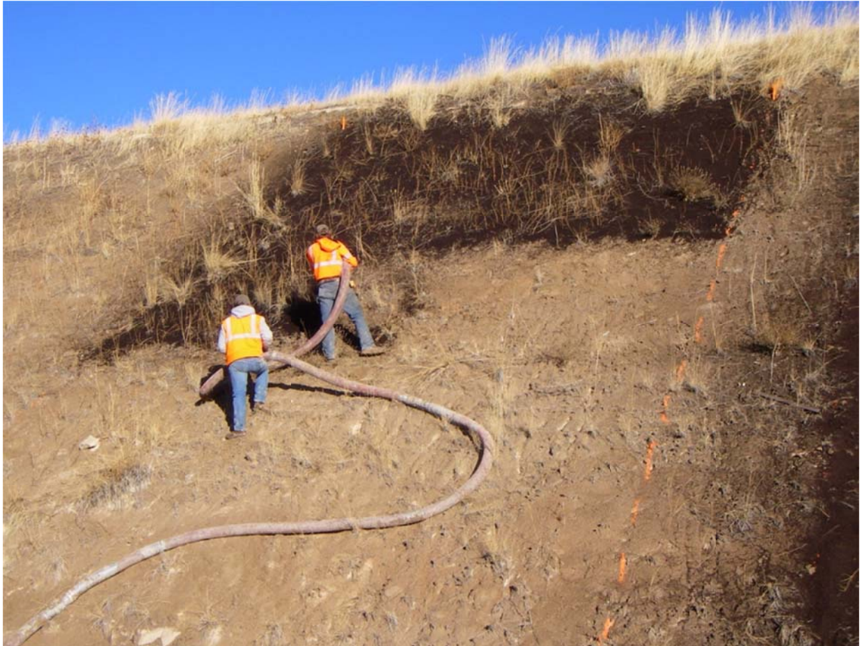
Figure 7: Application of compost on a test plot using a blower truck.
