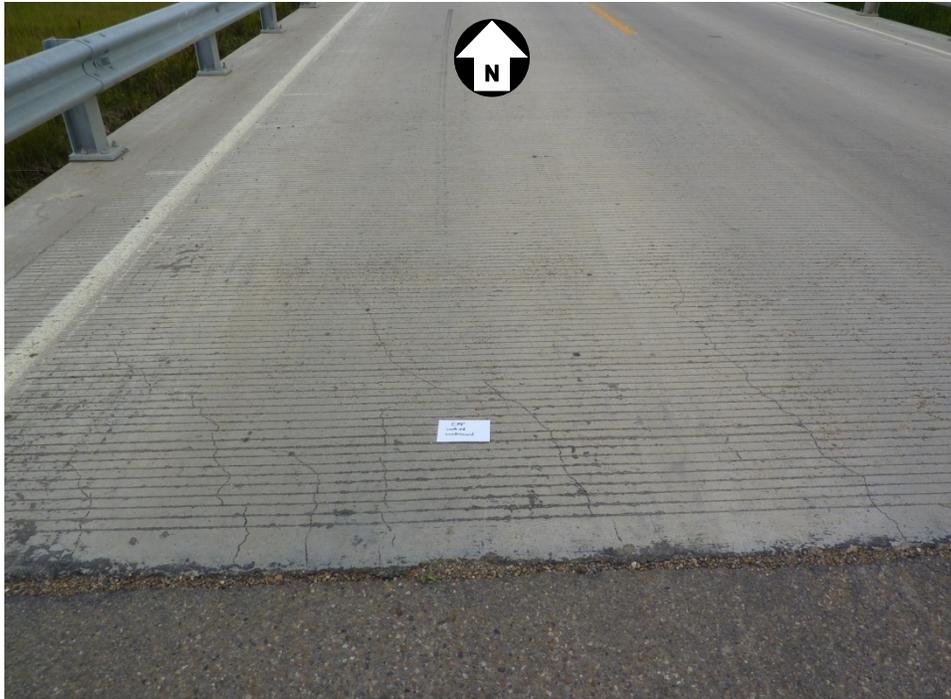
**Figure 14: Cracking on the southwest end of the Empirical deck in 2009.**
