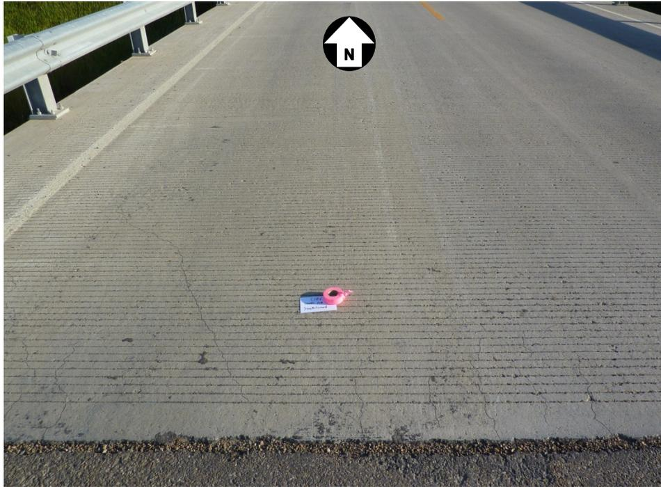
**Figure 13: Cracking on the southwest end of the Conventional deck in 2009.**
