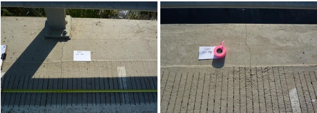
**Figure 15: Cantilever edge cracking, eastern edge, HPC–left, Conventional–right, in 2009.**
