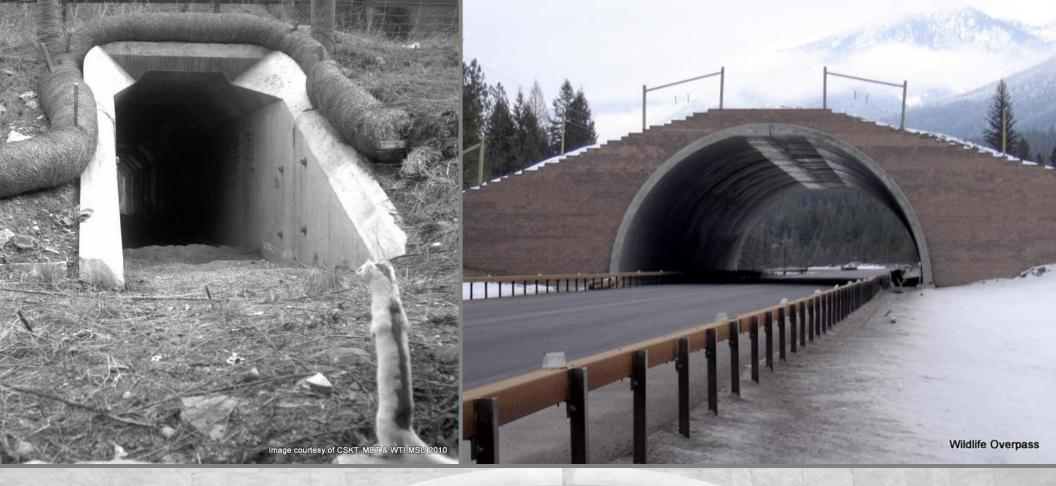
Mitigation measures include 41 fish and wildlife-crossing structures: 40 underpasses of various dimensions and types, and one overpass.
