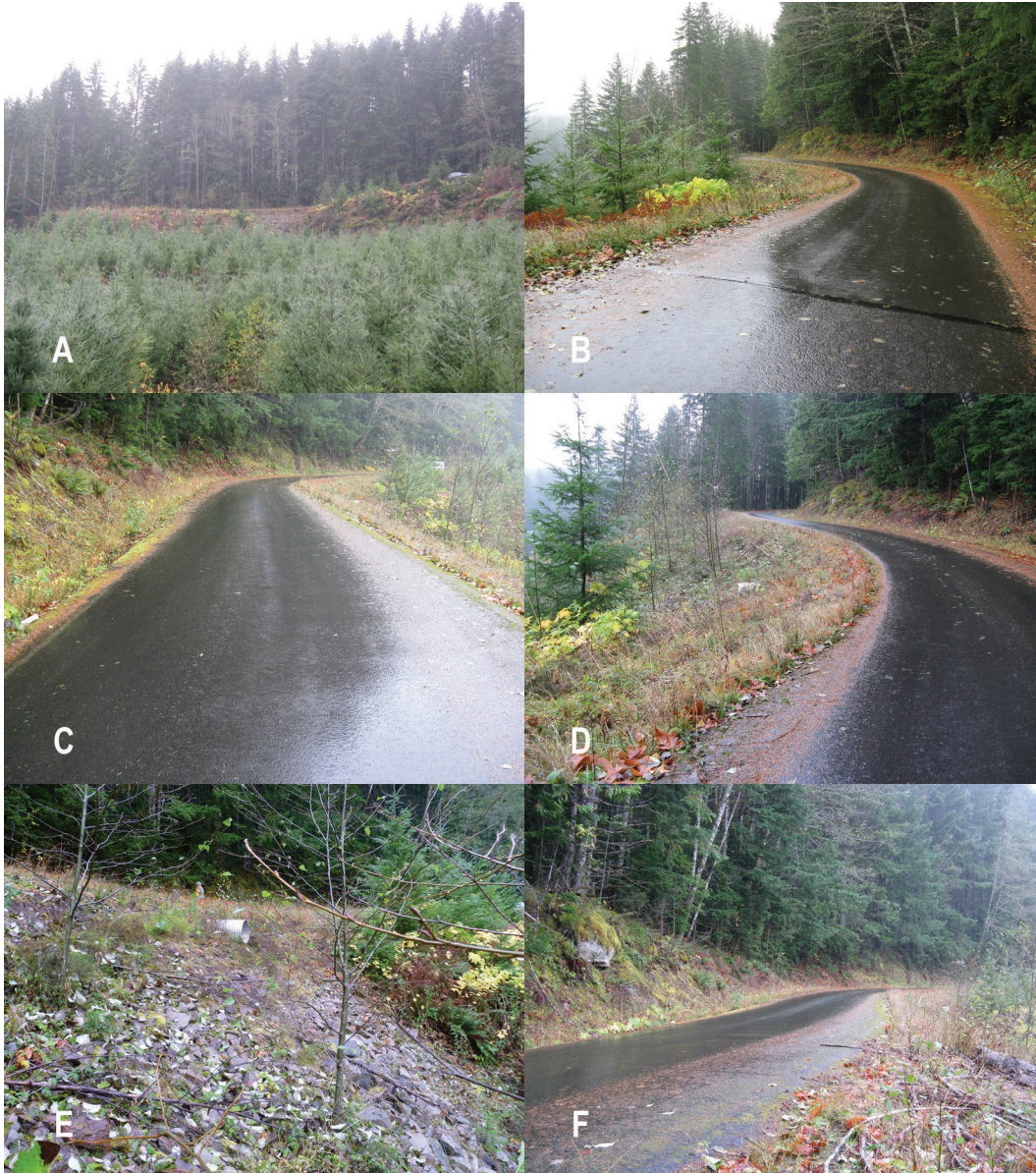
Figure 11: Photos of Road 26, Gifford Pinchot National Forest, MP 1.1 a) distant view of site from lower road, b) layout of site from end of repair, c) road surface, d) road surface with fill slope, e) fill slope showing drainage features and protective stone facing, and f) road surface with cut slope.
