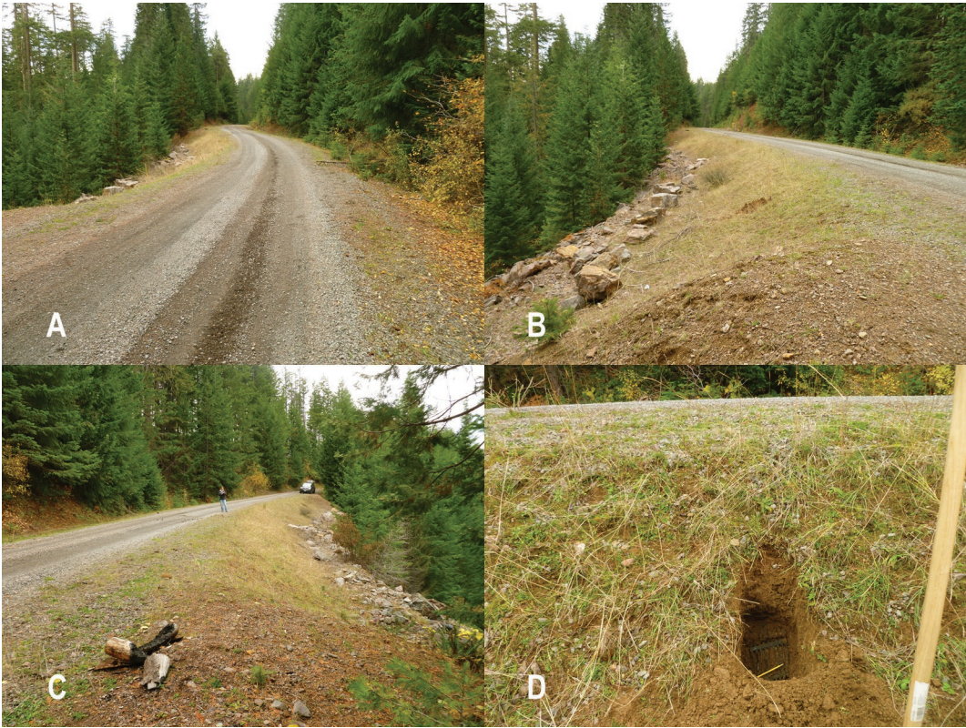
Figure 45: Photos of deep patch repairs at Site 3 on Road 6610, Rogue River-Siskiyou National Forest showing a) layout of site and road surface, b) layout of site and embankment, c) layout of site and embankment from the other end, d) geogrid reinforcement in embankment.
