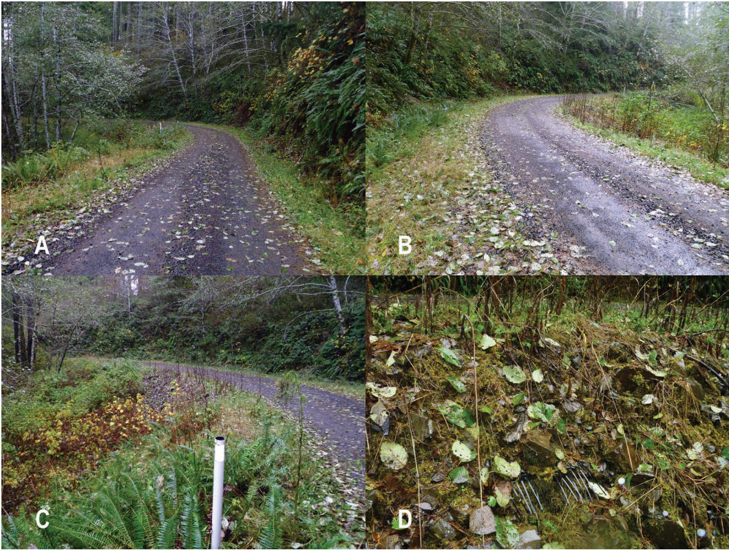
Figure 31: Photos of deep patch repairs on Road 58, Siuslaw National Forest a) layout of site from end of repair, b) layout of site looking from other end, c) fill slope showing stone facing, and d) close-up of deep patch showing exposed geogrid.
