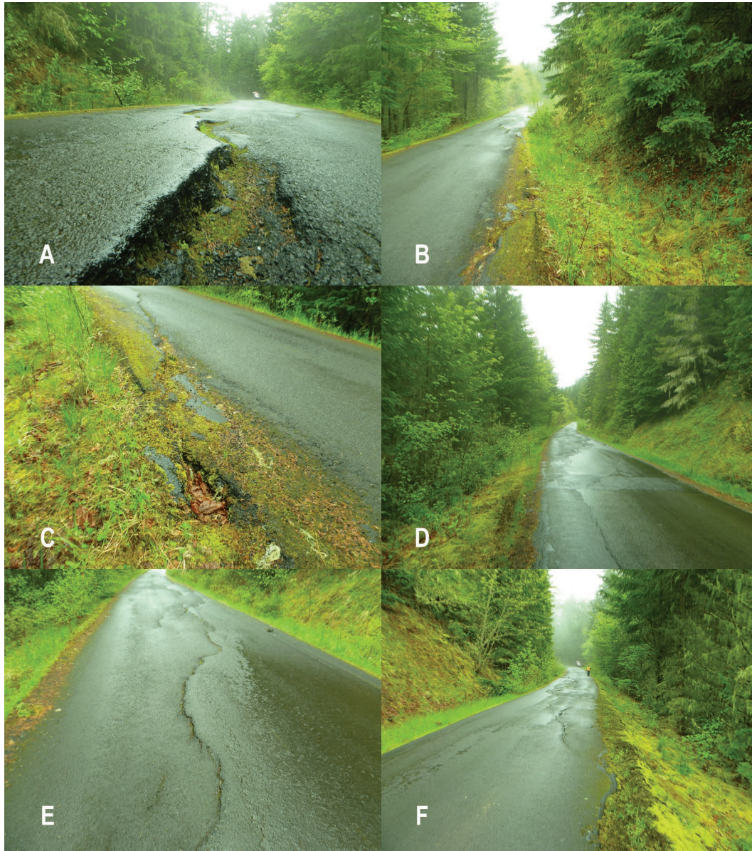
Figure 26: Photos of distresses on Road 45, Mount Hood National Forest, MP 28.2 a) close-up of differential settlement at crack interface, b) crack extending to inside shoulder, c) close-up of crack at inside shoulder, d) general view of road surface distresses, e) surface cracking and f) general view of surface distresses.
