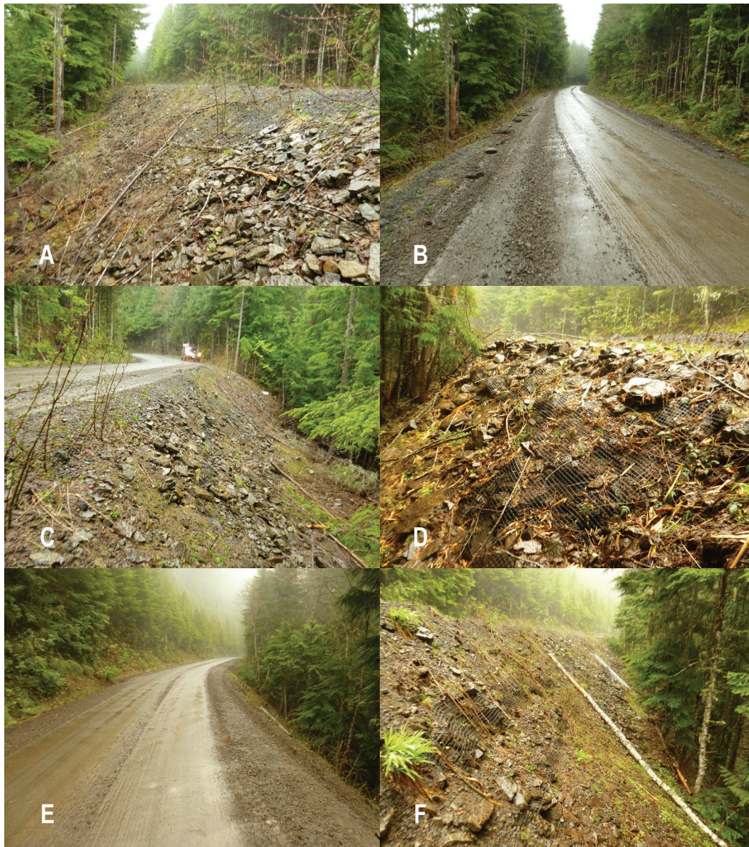
Figure 23: Photos of Road 45, Mount Hood National Forest, deep patch repairs at MP 5.85 (a, b, c) and MP 6.76 (d, e, f).
