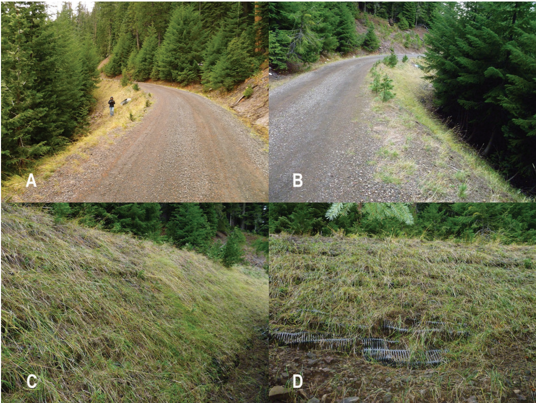
Figure 47: Photos of deep patch repairs at Site 12 on Road 6520, Rogue River-Siskiyou National Forest showing a) general layout of site and road surface, b) layout of site from other direction, c) embankment, d) exposed geogrid reinforcement in embankment.
