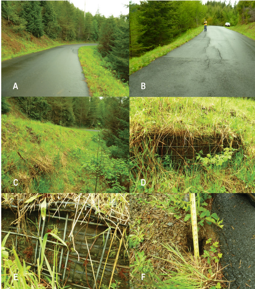
Figure 35: Photos of deep patch repairs at milepost 7.92 on Road 17, Siuslaw National Forest showing a) layout of site from end of repair, b) layout of site looking from other end, c) fill slope showing vertical facing, d) welded wire mesh to provide vertical support of slope face, e) close-up of vertical wire mesh showing geosynthetic reinforcement and separation geotextile, and f) hole near outside edge of pavement.
