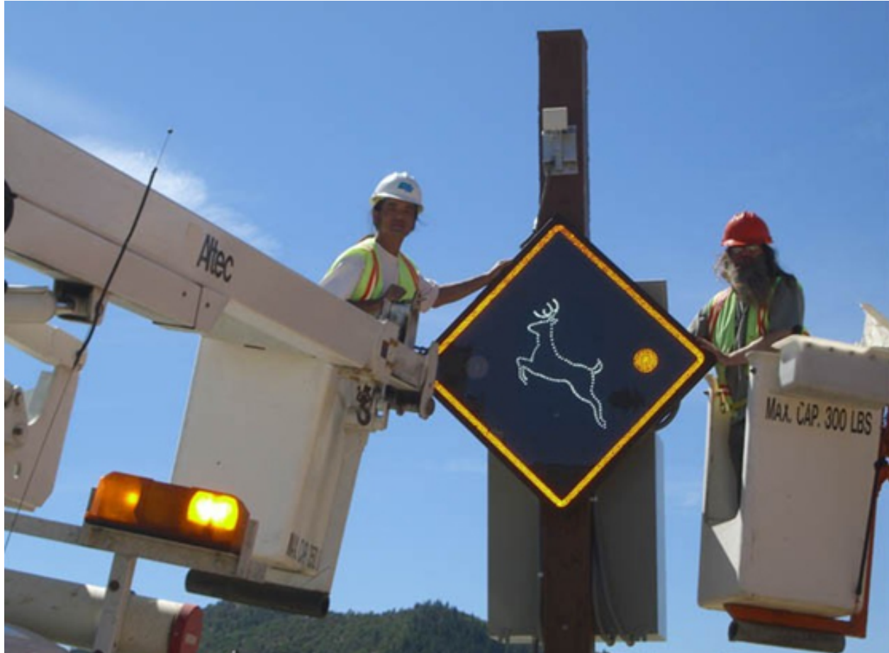
Figure 3.3: Installation of an Animal Warning Sign.
