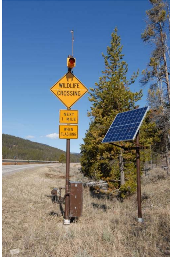
Figure 47. An animal detection system (microwave radio signal break-the-beam system manufactured by Sensor Technologies & Systems, Scottsdale, AZ) installed along a 1 mile (1,609 m) section of US Hwy 191 between Big Sky and West Yellowstone in Yellowstone National Park (© Marcel Huijser).
