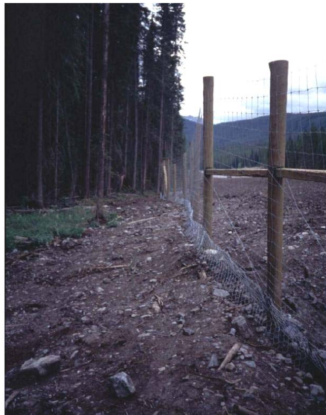
Figure 22. A 2.4 m high fence with buried apron along the Trans-Canada Highway in Banff National Park (Phase 3-A) (© Tony Clevenger).
