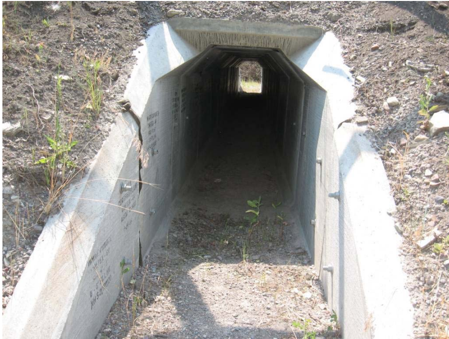
Figure 43. A medium mammal box culvert (1.2 m wide, 1.8 m high) along the 2-lane US Highway 93 on the Flathead Reservation in Montana, USA (south of Ravalli) (© Marcel Huijser).
