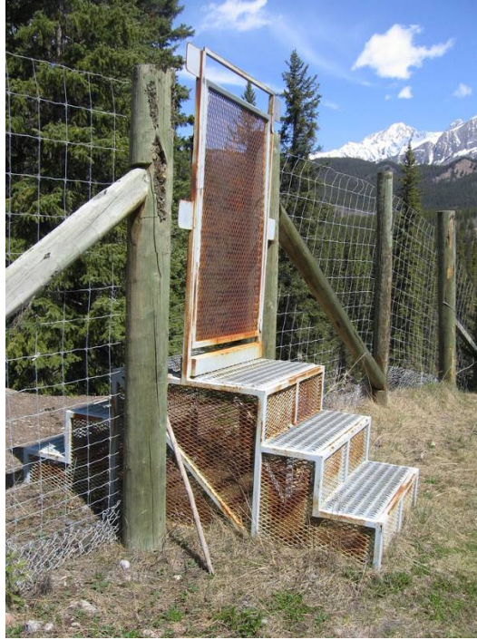
Figure 35: Swing gate in fence (spring loaded) allowing access for people, also when there is snow on the ground, along the Trans-Canada Highway in Banff National Park, Alberta, Canada (© Adam Ford, TCH research project / WTI-MSU).
