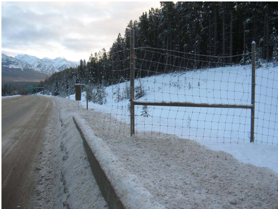
Figure 25. Fence end brought close to the road with a concrete barrier for safety along Hwy 93S in Banff National Park, just west of Castle Jct (© Marcel Huijser).
