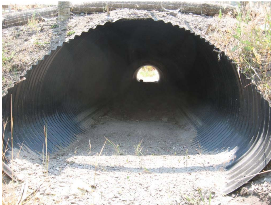
Figure 44. A medium mammal culvert (2 m wide, 1.5 m high) along the 2-lane US Highway 93 on the Flathead Reservation in Montana, USA (south of Ravalli) (© Marcel Huijser).
