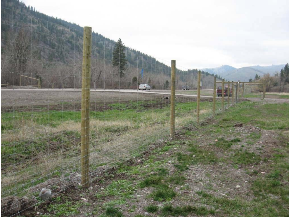
Figure 23. A 2.4 m high wildlife fence along the 2-lane US Highway 93 on the Flathead Reservation in Montana, USA (© Marcel Huijser).
