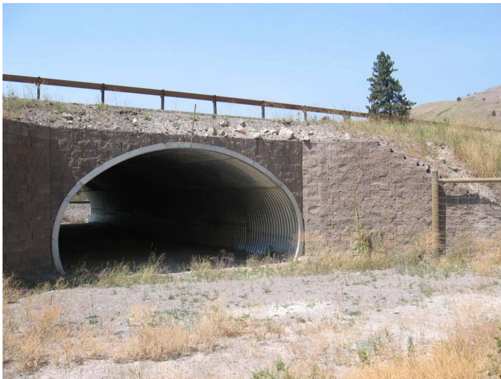
Figure 42. A large mammal underpass (7-8 m wide, 4-5 m high) along the 2-lane US Highway 93 on the Flathead Reservation in Montana, USA (south of Ravalli) (© Marcel Huijser).
