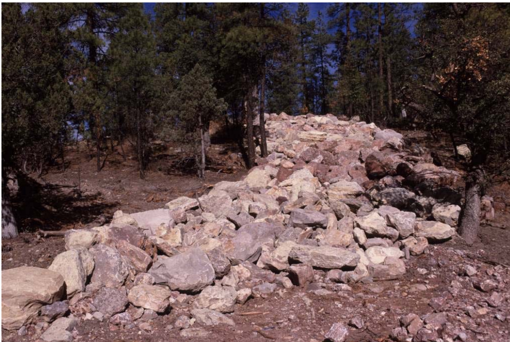
Figure 24. Large boulders placed in the right-of-way as a barrier to elk and deer along State Route 260 in Arizona, USA (© Marcel Huijser).
