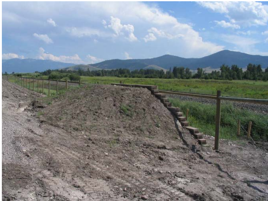
Figure 28. A jump-out along a 2.4 m (8 ft) high fence along US 93 in Montana, USA (© Marcel Huijser).
