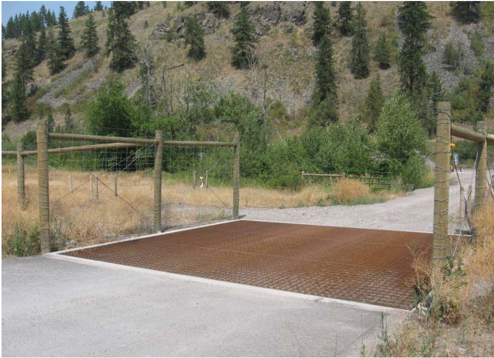
Figure 31. A wildlife guard at an access road of the 2-lane US Highway 93 on the Flathead Reservation in Montana, USA (© Marcel Huijser)
