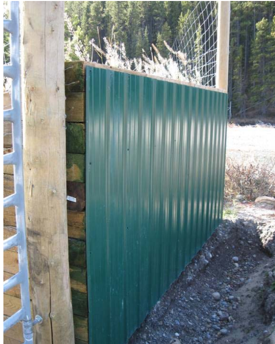
Figure 30. A jump-out along a 2.4 m (8 ft) high fence with smooth metal to prevent bears from climbing the jump-out the wrong way, along the Trans-Canada Highway, Lake Louise area, Banff National Park, Canada (© Marcel Huijser).
