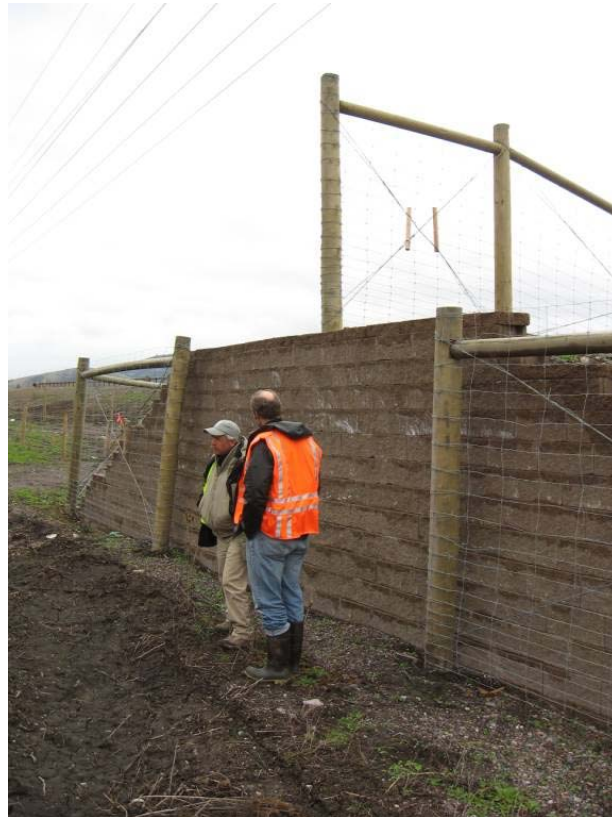
Figure 29. A jump-out along a 2.4 m (8 ft) high fence along US 93 in Montana, USA (© Marcel Huijser).
