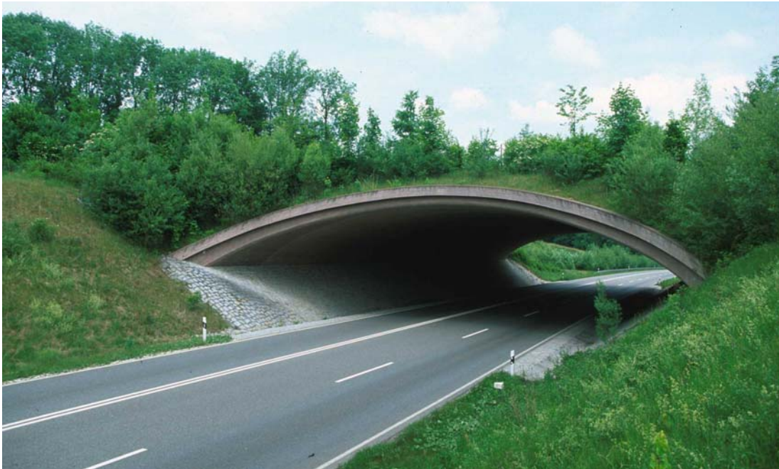
Figure 40. Wildlife overpass ("Schwarzgraben") across a 2-lane road (B31) in southern Germany (© Edgar van der Grift).
