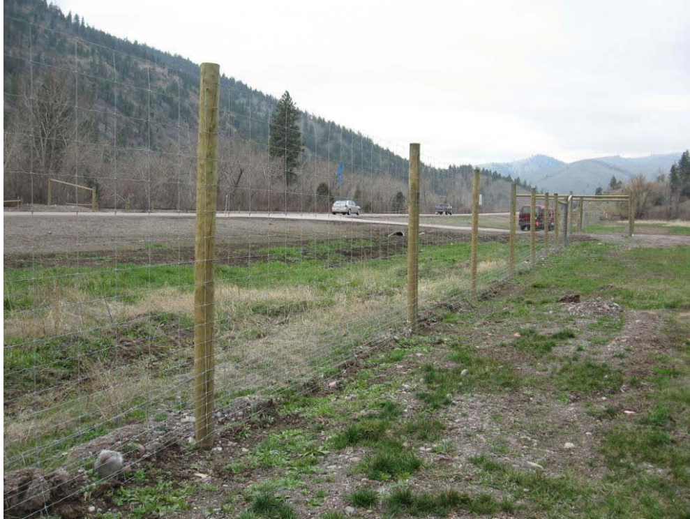
Figure 26. A 2.4 m high wildlife fence along the 2-lane US Highway 93 on the Flathead Reservation in Montana, USA (© Marcel Huijser).
