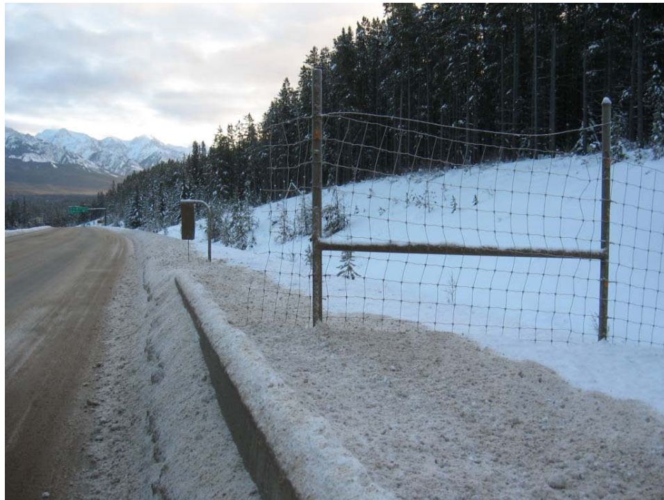
Figure 28. Fence end brought close to the road with a concrete barrier for safety along Hwy 93S in Banff National Park, just west of Castle Jct (© Marcel Huijser).
