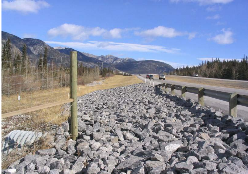
Figure 29. The Boulder Field at the Fence End at Dead Man's Flats Along the Trans Canada Highway East of Canmore, Alberta, Canada (© Bruce Leeson).
