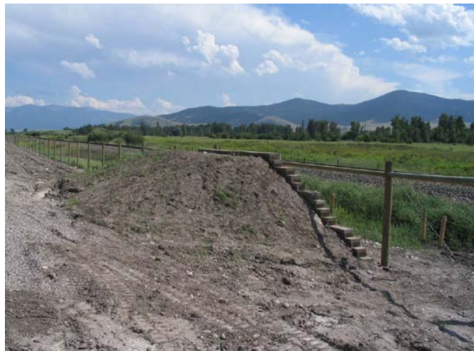
Figure 31. A jump-out along a 2.4 m (8 ft) high fence along US 93 in Montana, USA (© Marcel Huijser).
