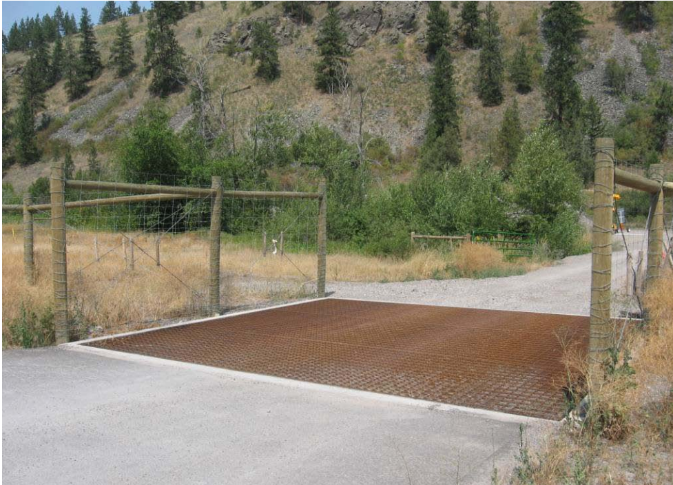
Figure 34. A wildlife guard at an access road of the 2-lane US Highway 93 on the Flathead Reservation in Montana, USA (© Marcel Huijser).
