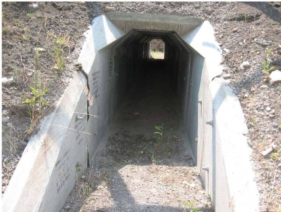
Figure 46. A medium mammal box culvert (1.2 m wide, 1.8 m high) along the 2-lane US Highway 93 on the Flathead Reservation in Montana, USA (south of Ravalli) (© Marcel Huijser).
