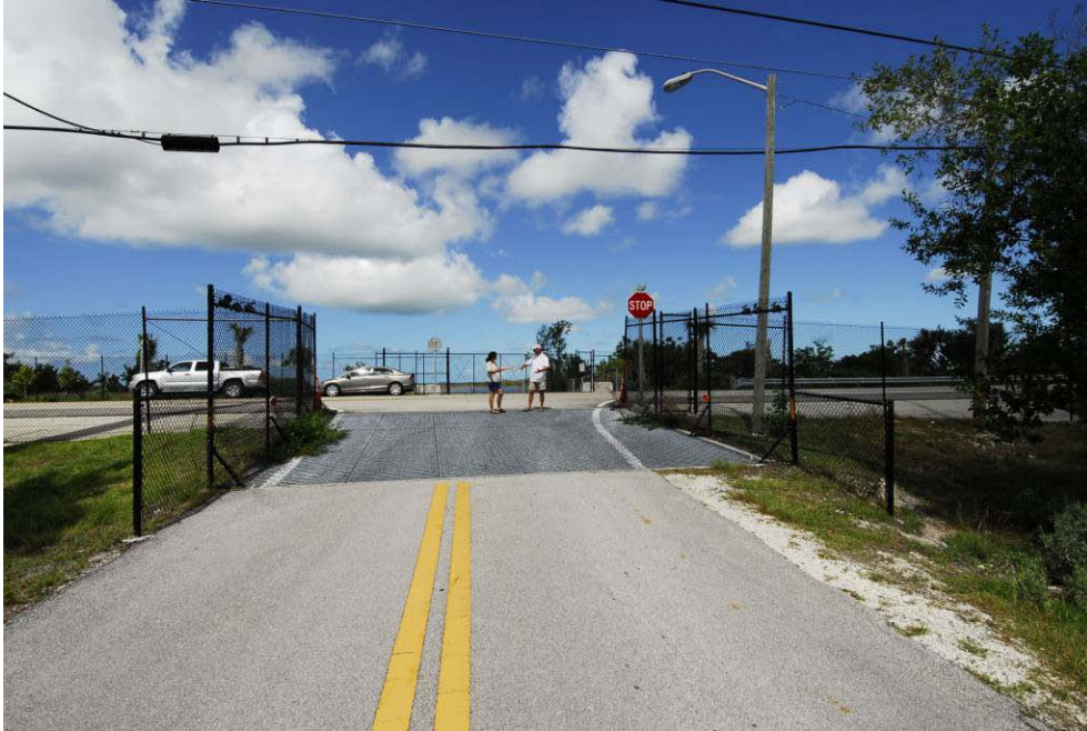
Figure 35. A wildlife guard at an access road of the 2-lane US Highway 1 on Big Pine Key, Florida, USA (© Marcel Huijser).
