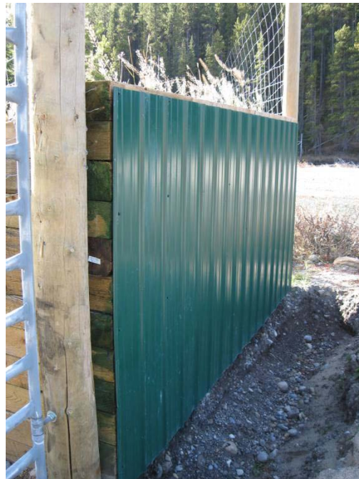
Figure 33. A jump-out along a 2.4 m (8 ft) high fence with smooth metal to prevent bears from climbing the jump-out the wrong way. Along the Trans Canada Highway, Lake Louise area, Banff National Park, Canada (© Marcel Huijser).
