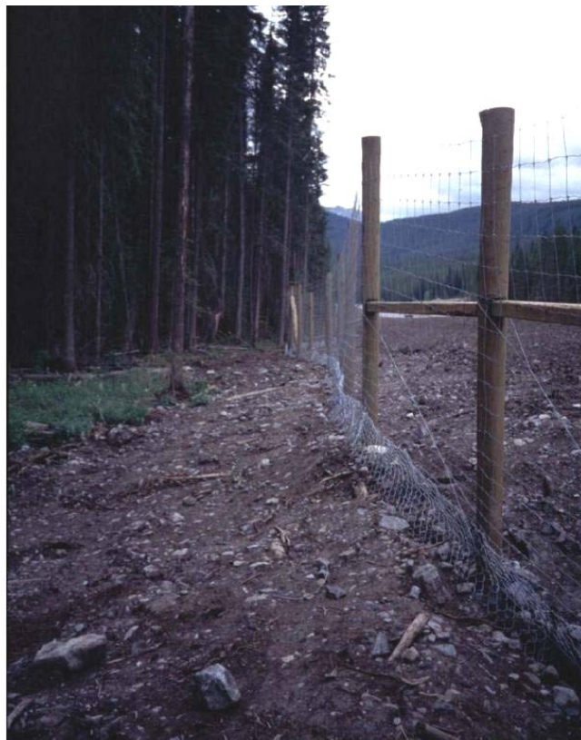
Figure 25. A 2.4 m high fence with buried apron along the Trans-Canada Highway in Banff National Park (Phase 3-A) (© Tony Clevenger).
