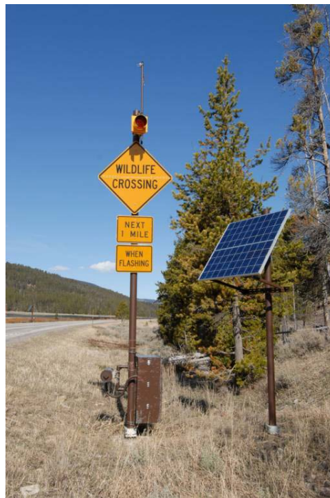
Figure 50. An animal detection system (microwave radio signal break-the-beam system manufactured by Sensor Technologies & Systems, Scottsdale, AZ) installed along a 1 mile (1,609 m) section of US Hwy 191 between Big Sky and West Yellowstone in Yellowstone National Park (© Marcel Huijser).
