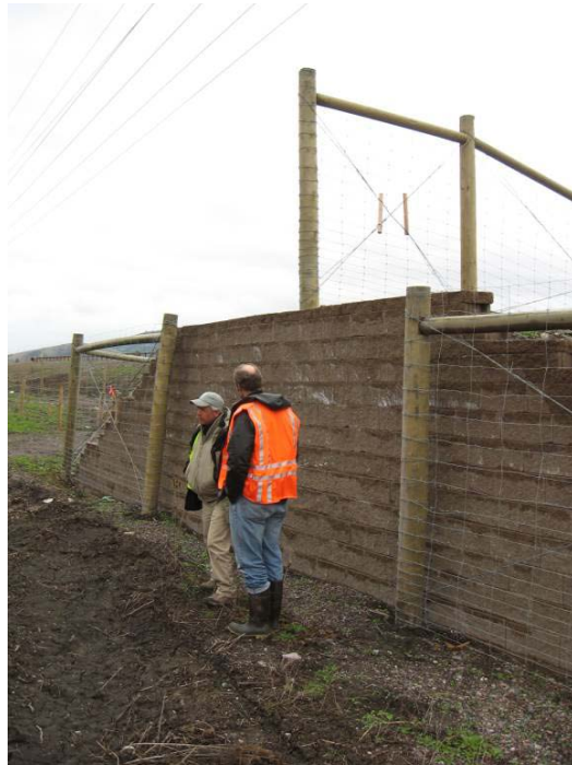
Figure 32. A jump-out along a 2.4 m (8 ft) high fence along US 93 in Montana, USA (© Marcel Huijser).
