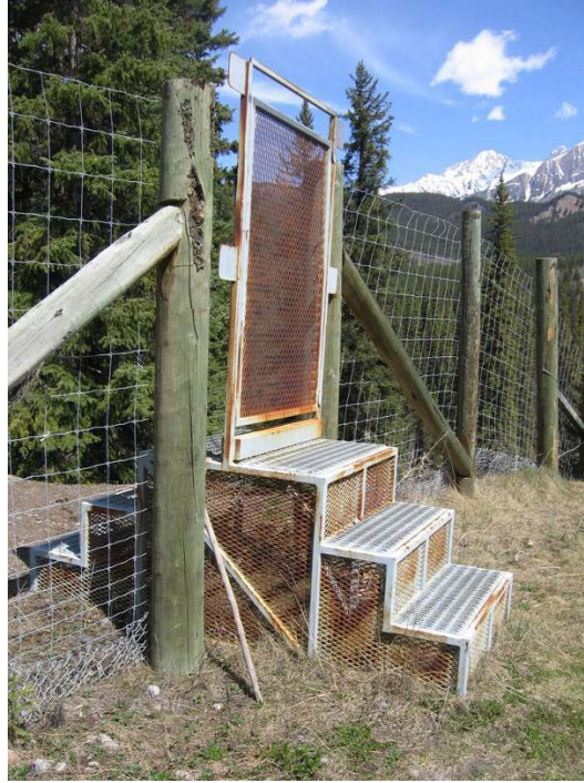
Figure 38: Swing gate in fence (spring loaded) allowing access for people, also when there is snow on the ground, along the Trans-Canada Highway in Banff National Park, Alberta, Canada (© Adam Ford, TCH research project / WTI-MSU).
