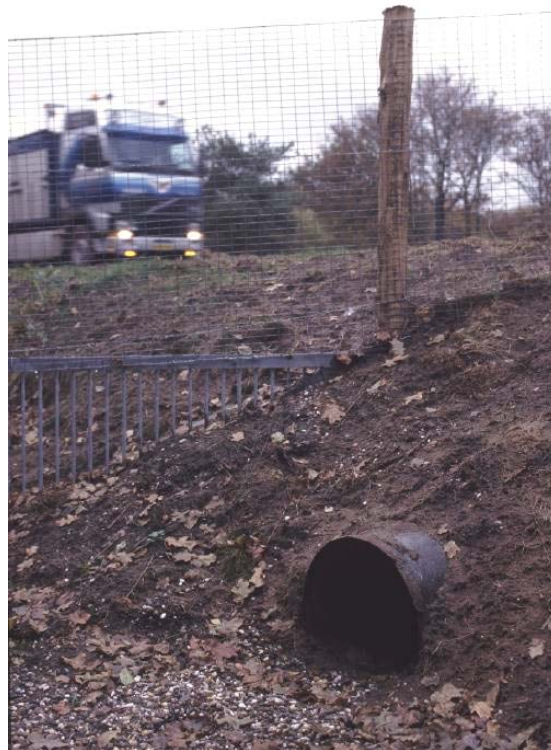
Figure 48. A small-medium mammal pipe (“badger pipe”) in The Netherlands (© Marcel Huijser).
