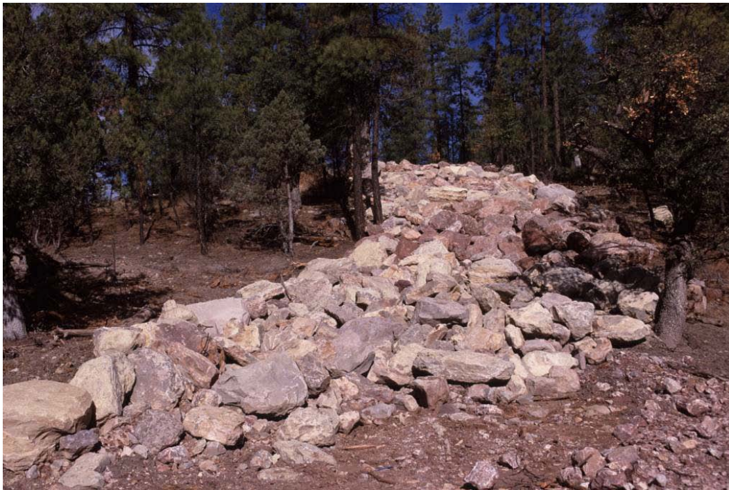
Figure 27. Large boulders placed in the right-of-way as a barrier to elk and deer along State Route 260 in Arizona, USA (© Marcel Huijser).
