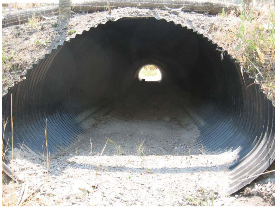
Figure 47. A medium mammal culvert (2 m wide, 1.5 m high) along the 2-lane US Highway 93 on the Flathead Reservation in Montana, USA (south of Ravalli) (© Marcel Huijser).
