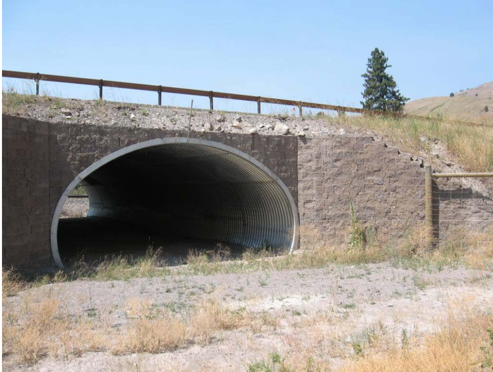
Figure 45. A large mammal underpass (7-8 m wide, 4-5 m high) along the 2-lane US Highway 93 on the Flathead Reservation in Montana, USA (south of Ravalli) (© Marcel Huijser).
