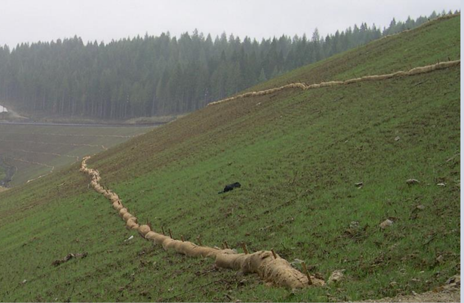
Figure 7. The combination of surface roughening, wattles, mulch, and seeding resulted in stable conditions at the Electrical Substation Site.
