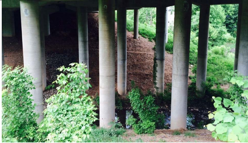
(b) South Side of Underpass
