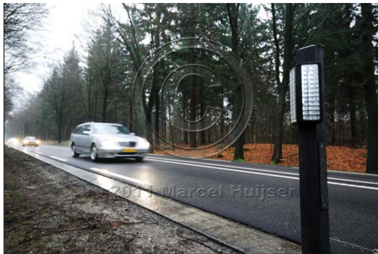
Figure 2-4 Wildlife Reflector Installed in Right-of-Way
