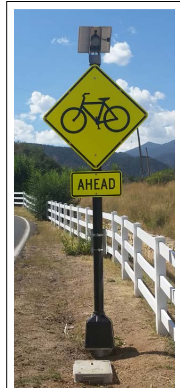
Photo of dynamic warning system in Colorado Springs
