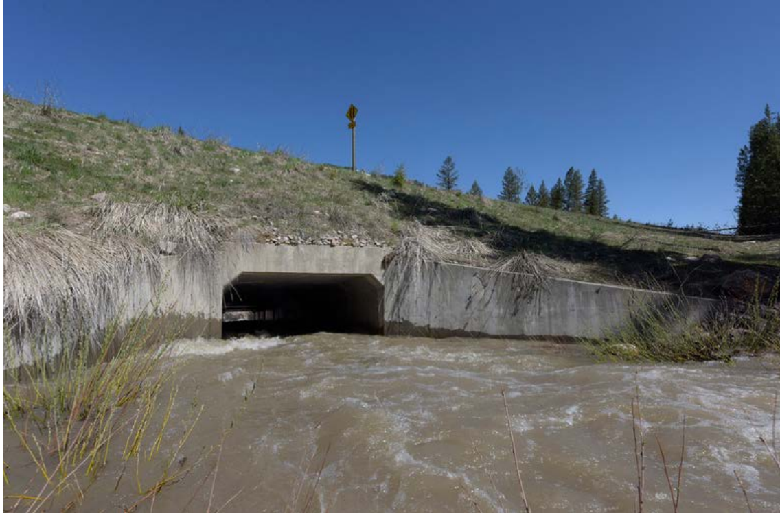
Figure 22. A box culvert (US Hwy 26.89, Cabin Creek).
