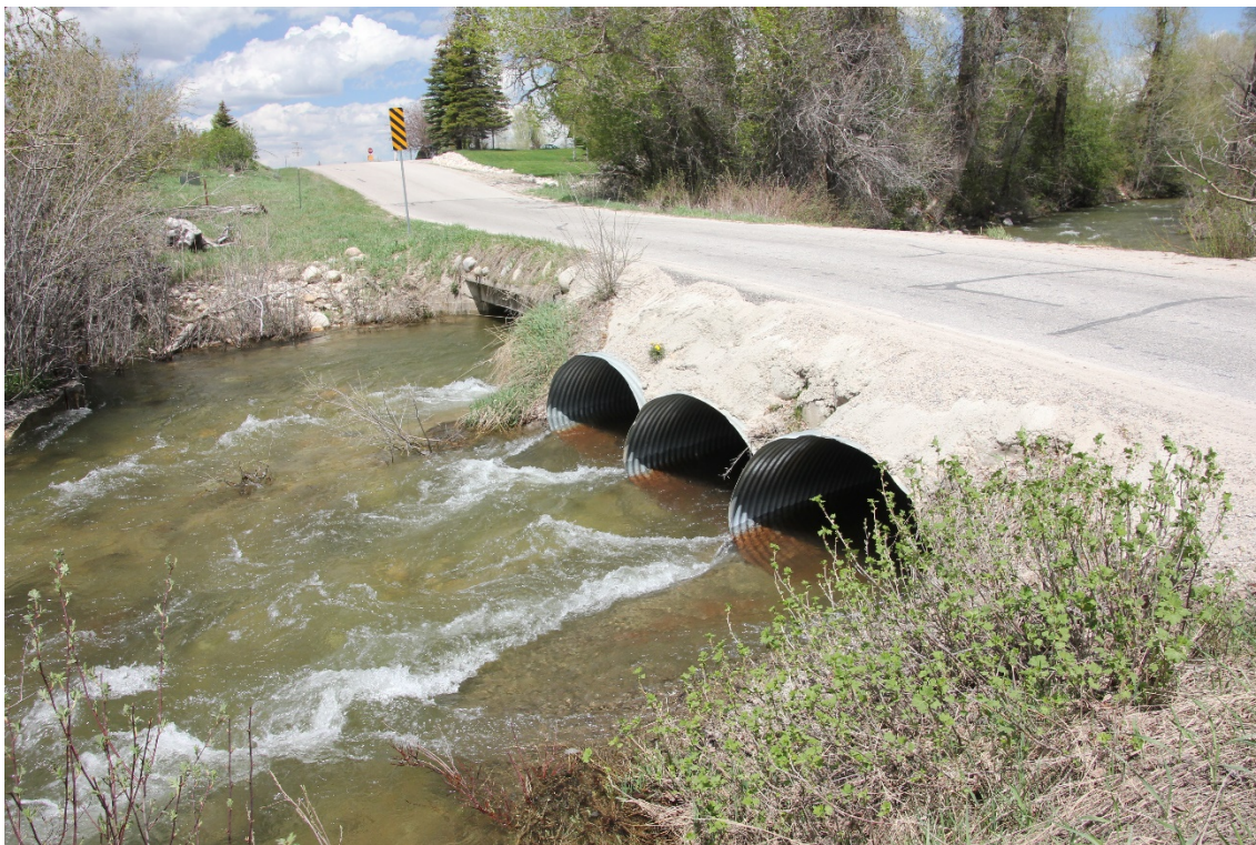
Figure 21. A multi-barrel crossing (site 65 along Stateline Rd, Teton Creek). View from downstream left-bank of the stream.
