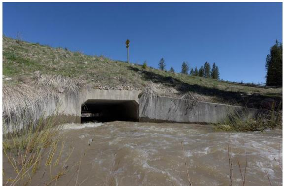
Figure 22. A box culvert (US Hwy 26.89, Cabin Creek).
