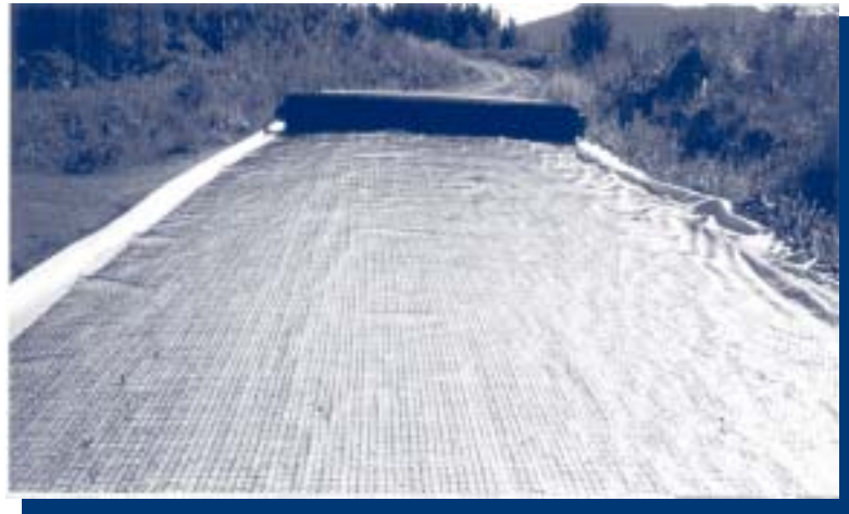
Above: A layer of reinforcement is added during road construction.
