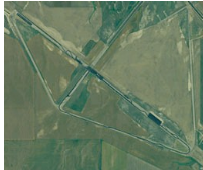
Aerial photo showing test tracks of TRANSCEND facility prior to construction and installation of snowmaking equipment, workshop, sub grade stabilization test strip and RADS test bed.
