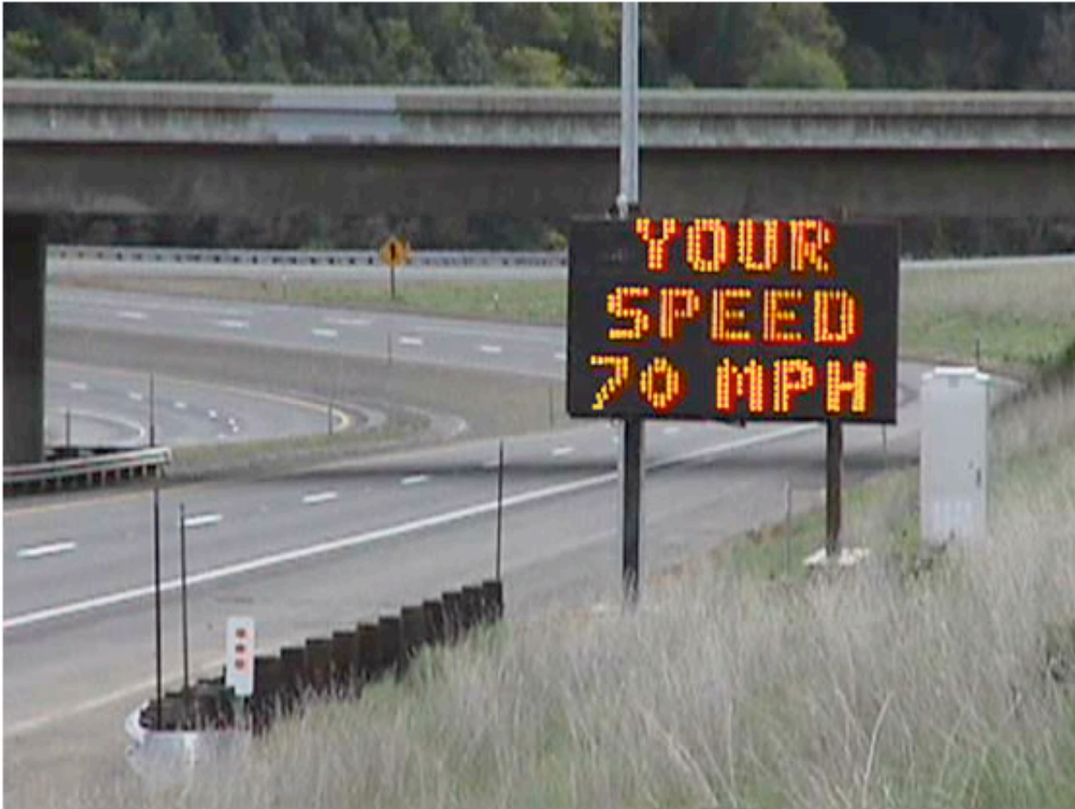
Curve warning system installation in Sacramento Canyon
