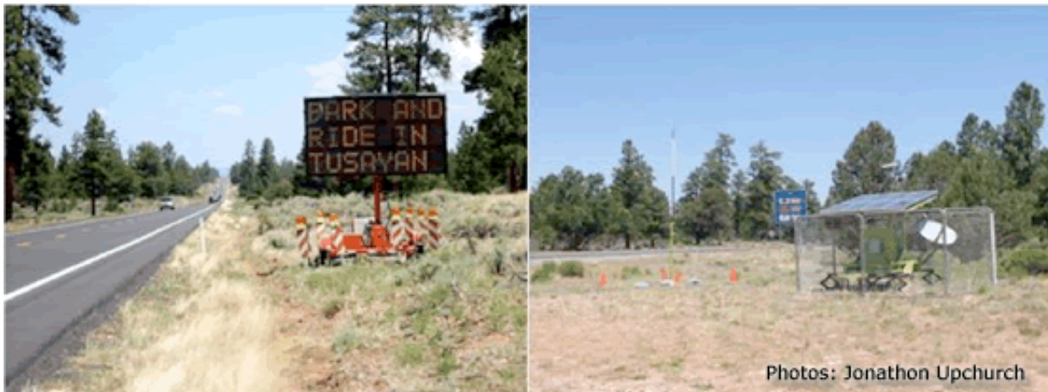
PDMS and HAR in the Gateway Community of Tusayan, used in tandem spaced approximately 2 miles apart
