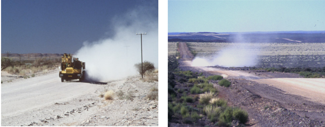
Figure 2: Fines lost from unsealed roads
