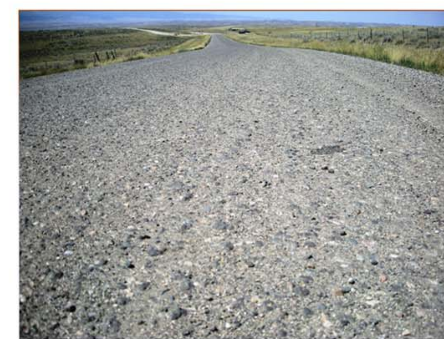
Blended RAP without CaCl three months after placement.
