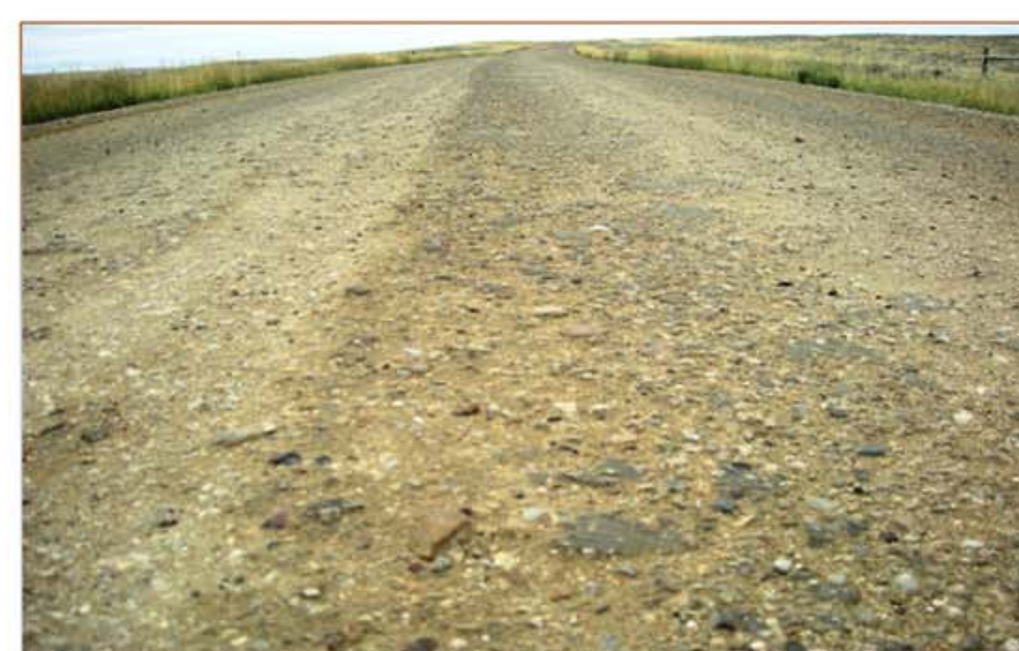
Schoonover Road section S0 aggregate control with CaCl three months after placement
