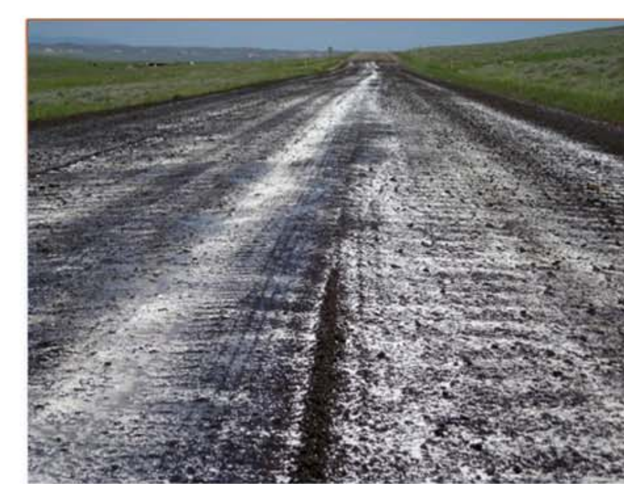
RAP blend sections with and without CaCl flakes. Water was applied, then flakes, then additional water.
