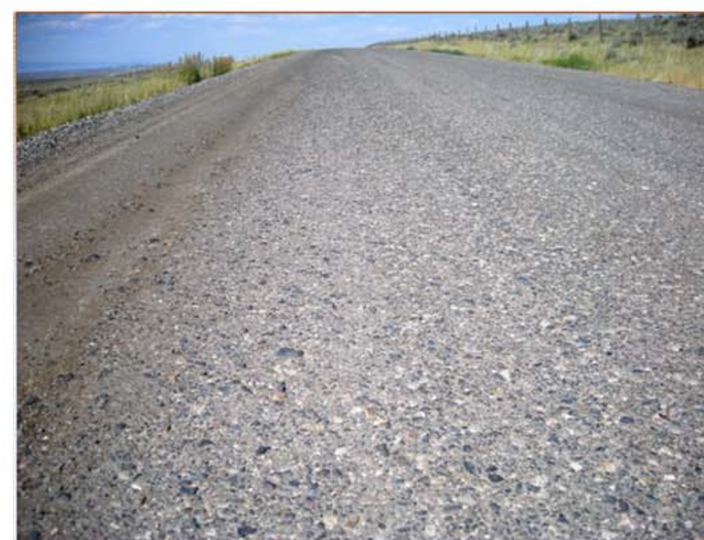
Blended RAP with CaCl three months after placement.
