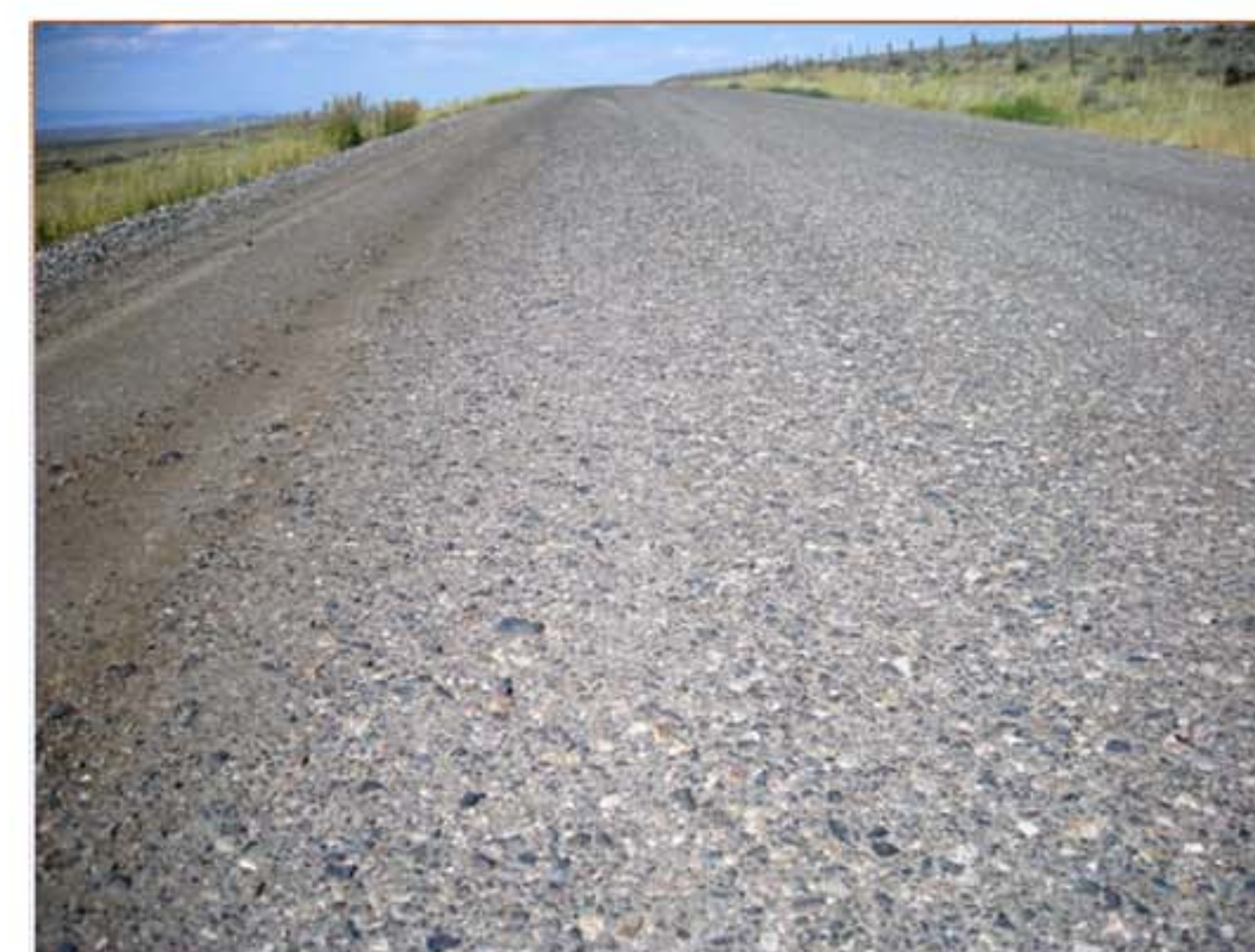
Blended RAP with CaCl three months after placement.
