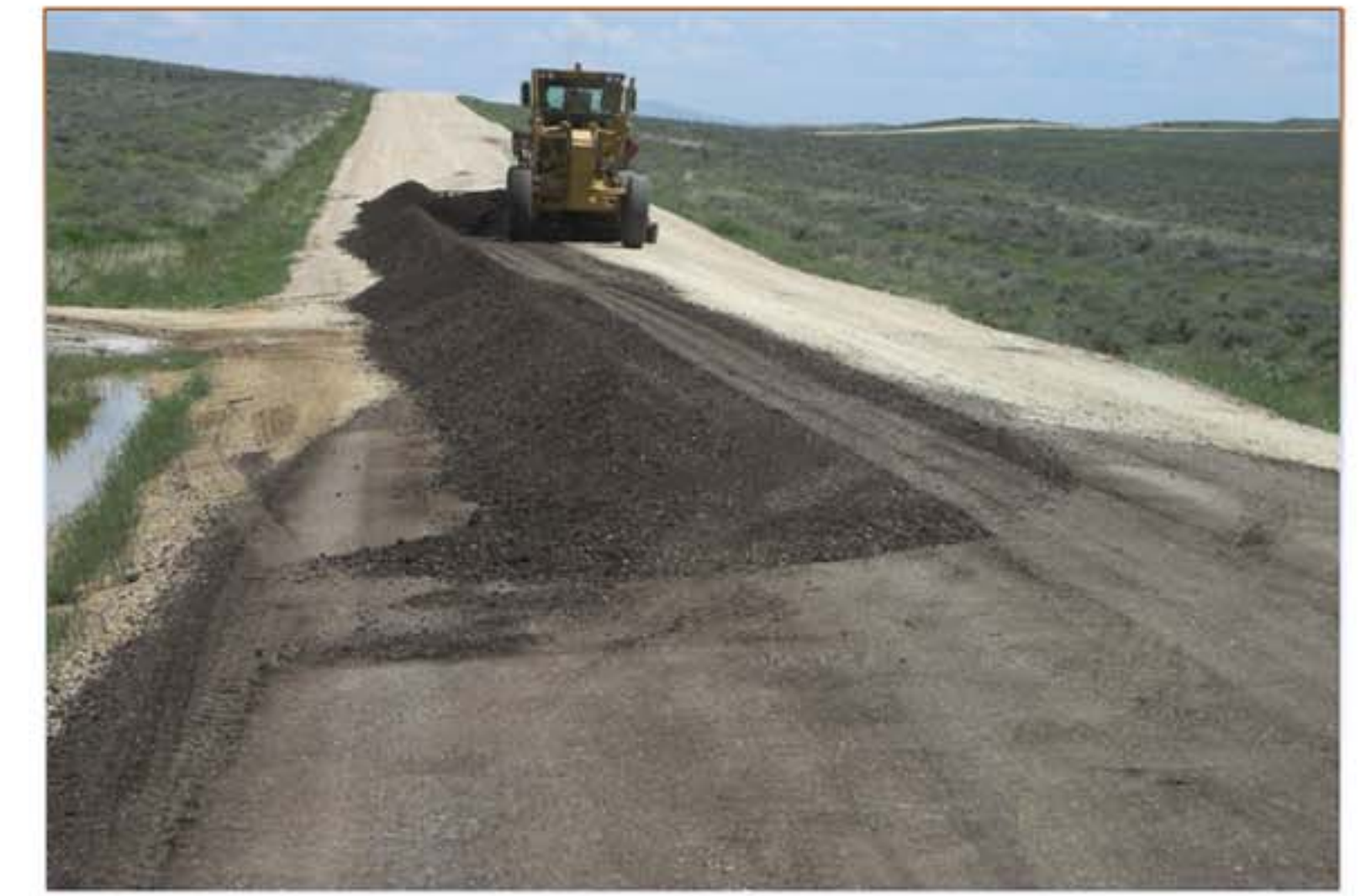
Spreading RAP and aggregate blend on Schoonover Road section S2.
