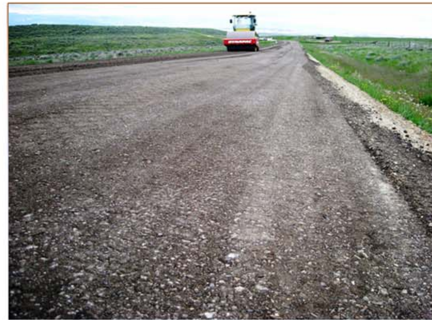
Compacted, pugmill blended RAP and aggregate on Schoonover Road.
