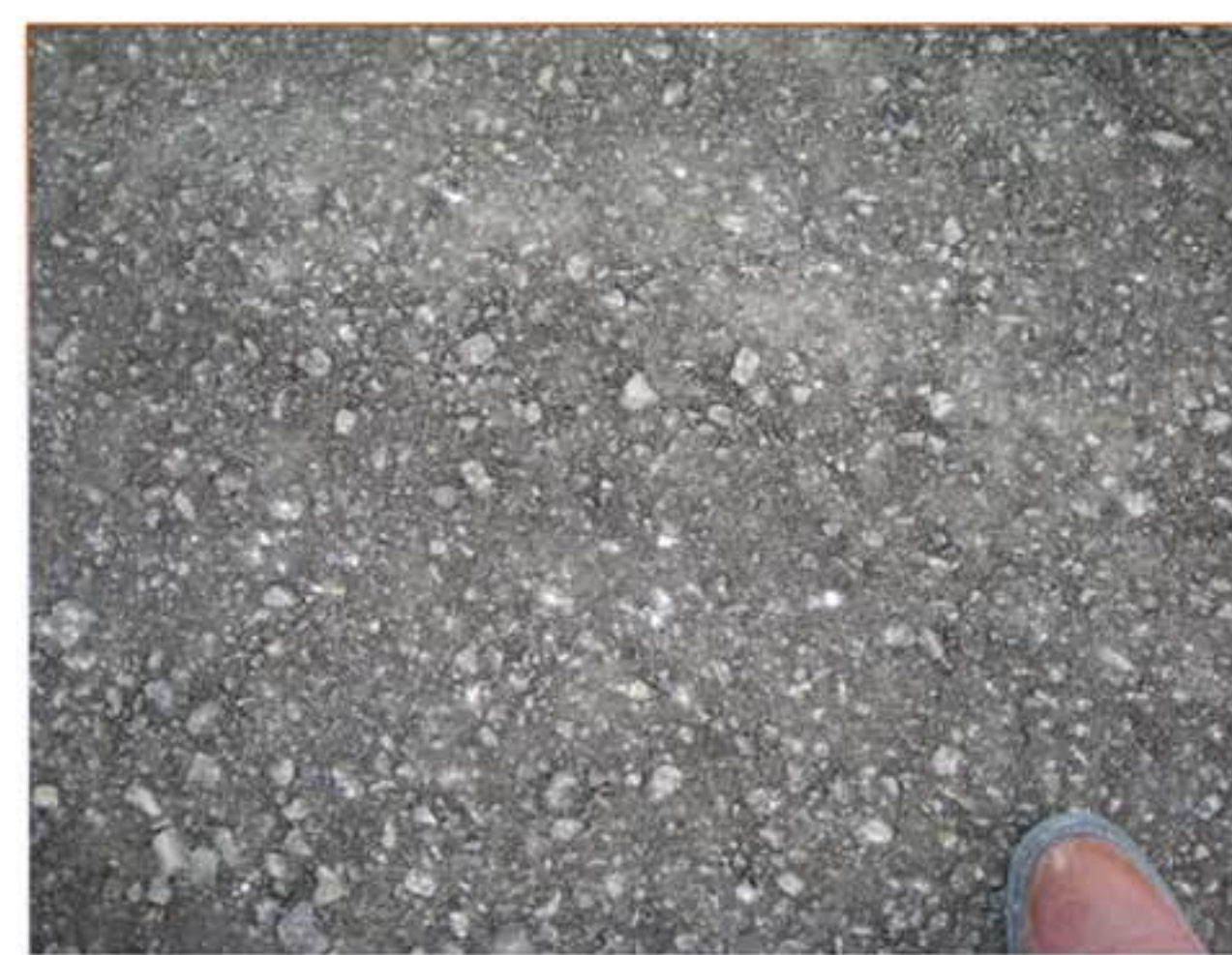
Compacted, pugmill blended RAP and aggregate on Schoonover Road.
