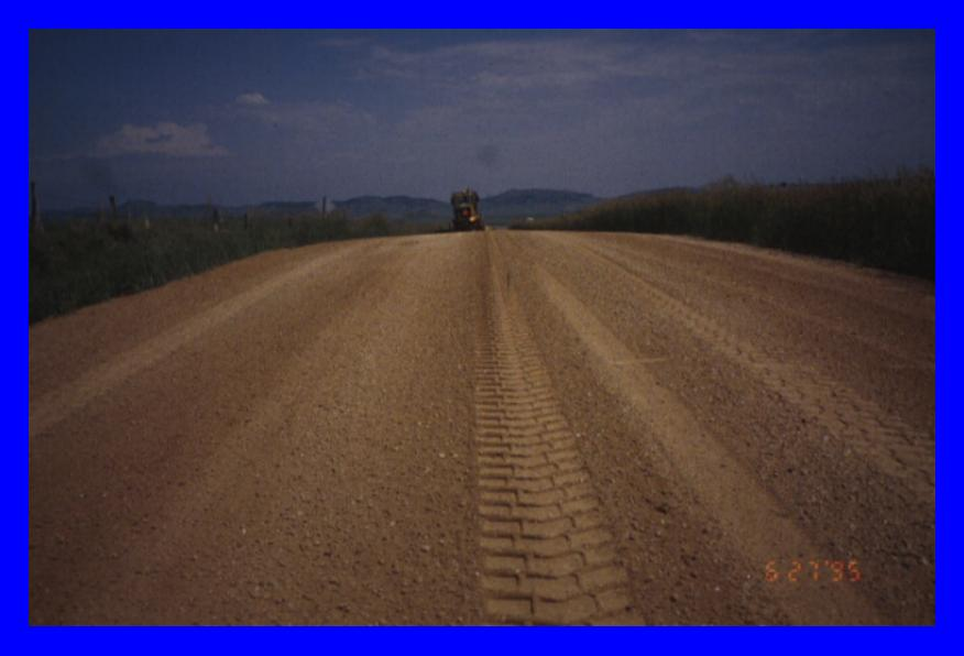
Very good crown, material nicely shaped with 1 to 2 inches of loose material.
