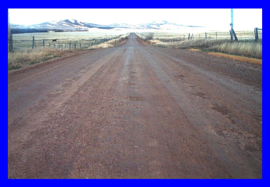
Good crown was never established, has poor drainage. Result is washboards and potholes.
