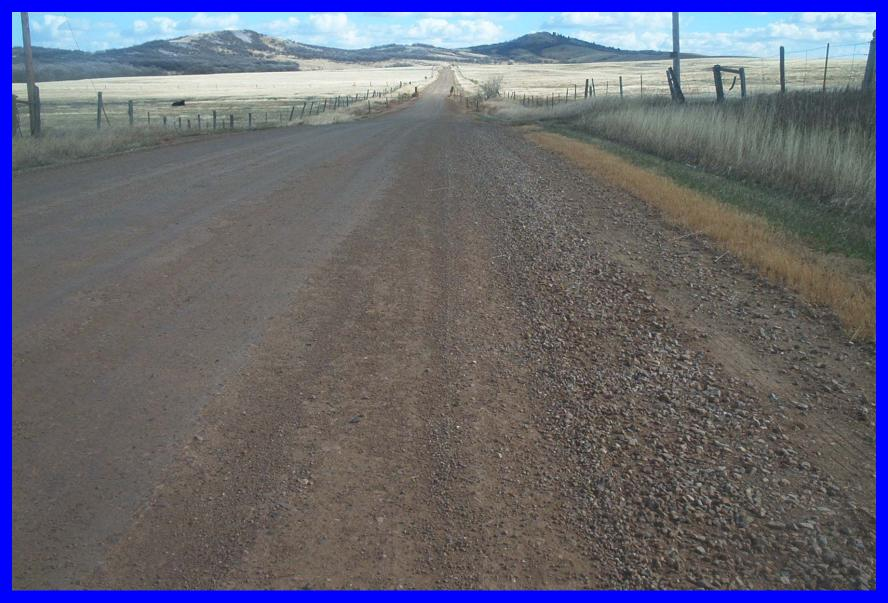
Uneven application of product results in failure at outside edge of roadway.
