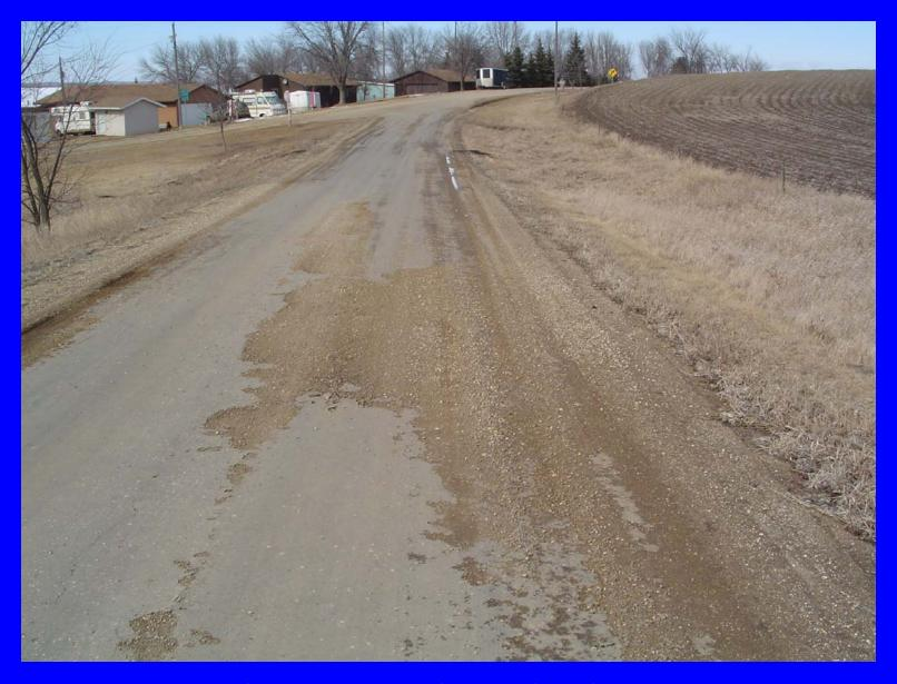
Poor penetration results in stripping and poor performance
