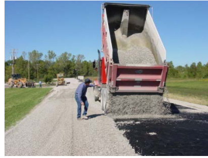
Figure 4. Surface layer placement (Photo Courtesy of John Bowders)
