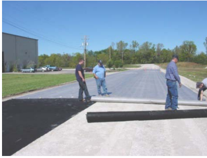
Figure 3. Geotextile layer installed prior to surfacing. (Photo courtesy of John Bowders)
