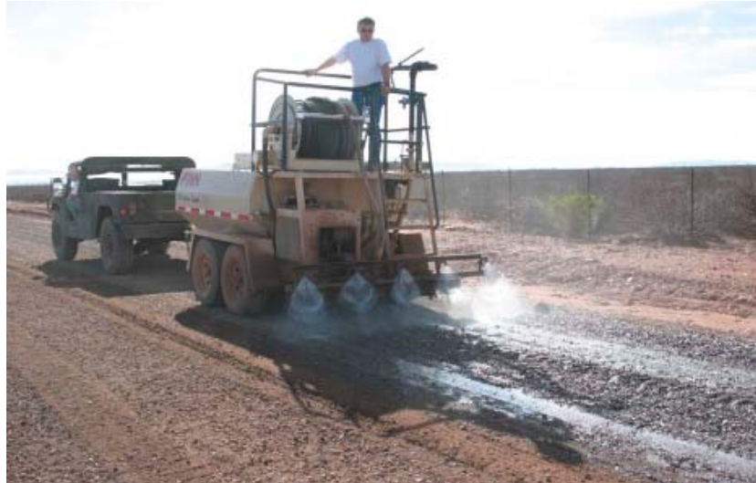
Figure 3. Treating road section in Douglas, AZ with chemical dust palliative.
