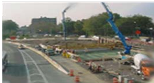
Work Zone Management
