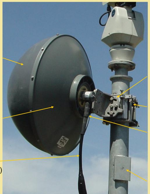
Antenna elevation adjustment
