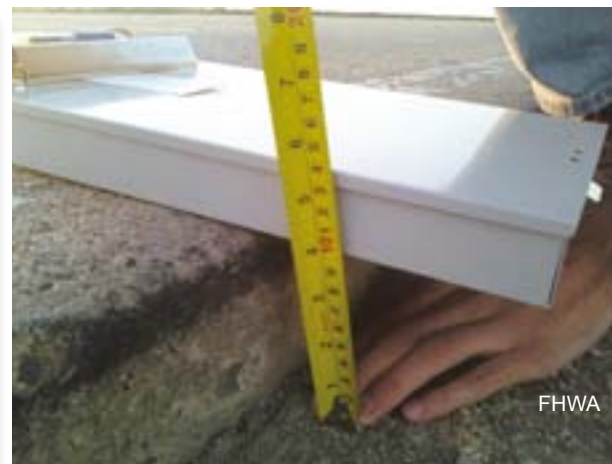
Pavement edge drop off creates a height differential which a vehicle must climb to overcome tire scrubbing. In the left photo, the drop off is at an isolated location that lacks vegetation. The photo on the right is a roadway with consistent drop offs due to farm equipment using the shoulder.
