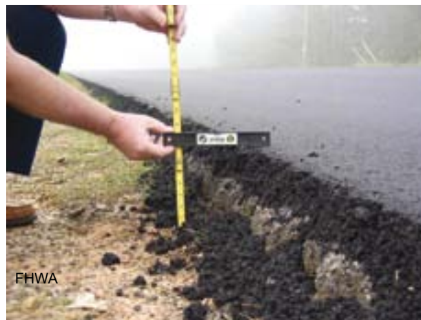
Pavement edge drop off creates a height differential which a vehicle must climb to overcome tire scrubbing. In the left photo, the drop off is at an isolated location that lacks vegetation. The photo on the right is a roadway with consistent drop offs due to farm equipment using the shoulder.
