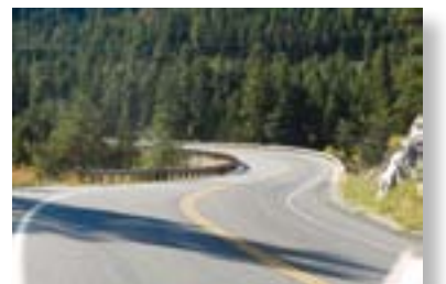
The cost of w-beam guardrail will vary regionally and over time. However, in-service studies reported a range of $11.44 per foot (2004) to $13.65 per foot (2003). 9,10 Adjusted to 2011 dollars, these figures would be $13.71 to $16.80, respectively. 11
