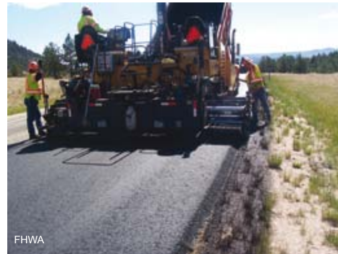
Installation of the Safety Edge SM coincides with the paving operation.
